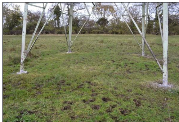
Figure 27. Base of Pylon FK10 without muffs
