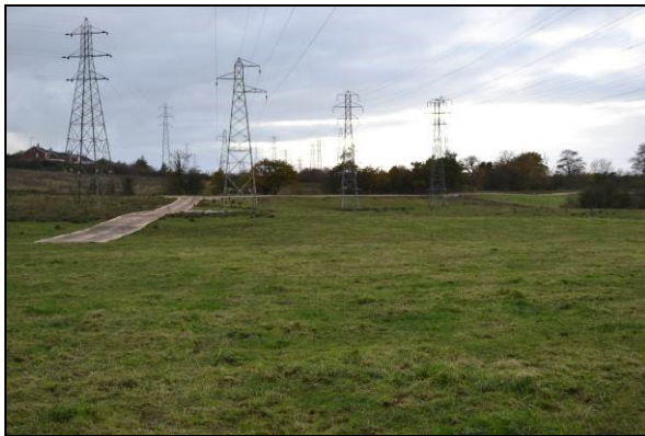
Figure 26. Mats leading to pylon FK10
