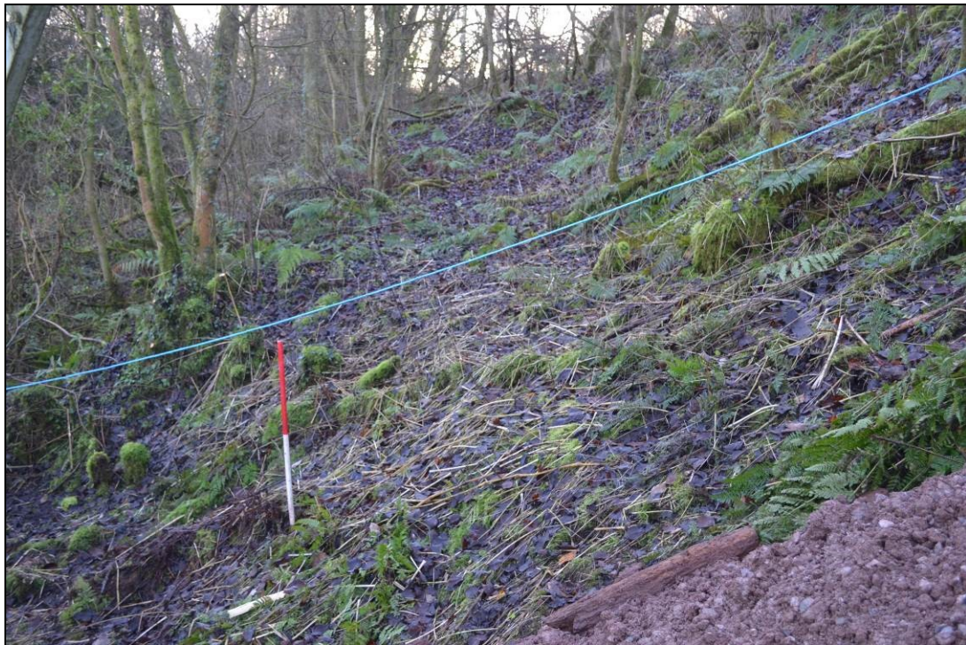
Figure 23 Ramp approaching Pylon FK5
