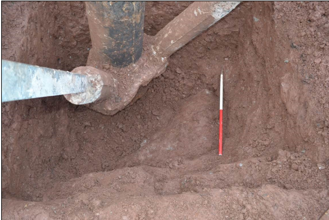
Figure 21. Final excavation of the western pylon leg
