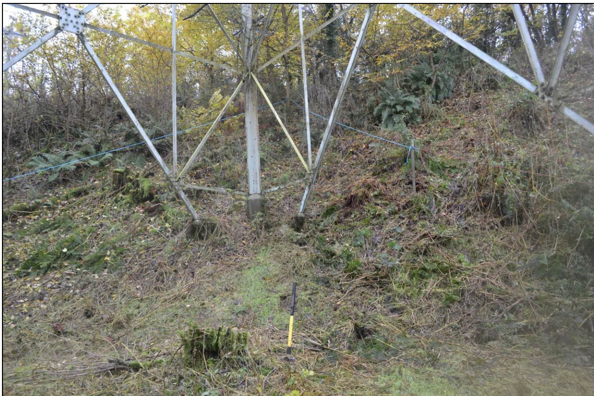
Figure 13. Western pylon leg prior to excavation
