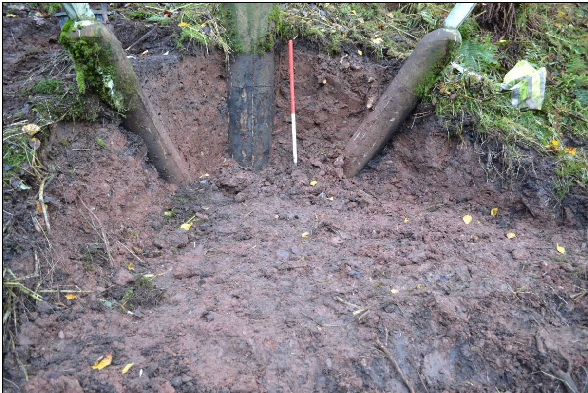
Figure 17. Initial removal of spoil beside the pylon
