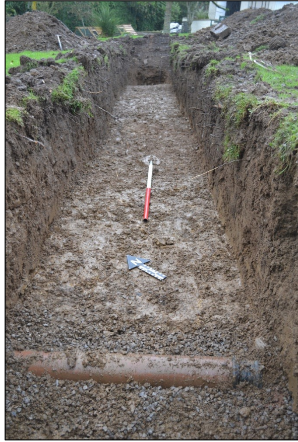
Figure 16. Upper portion of the trench
