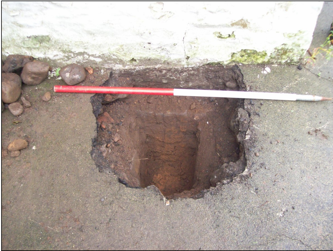
Figure 5. Reception pit for traffic sign
