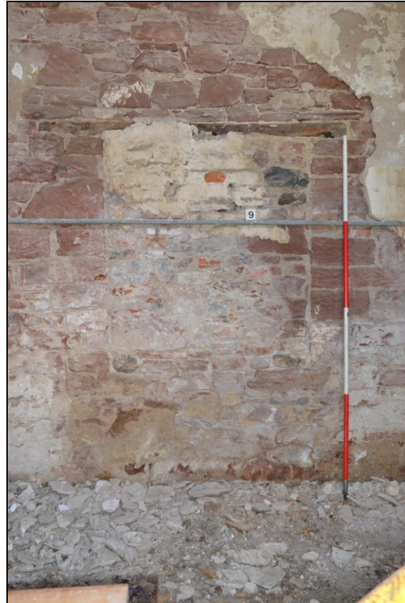
Figure 9. Filled window (9)
