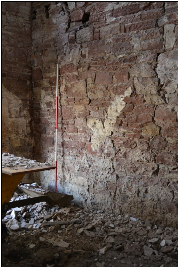
Figure 8. Interior of the cart shed
