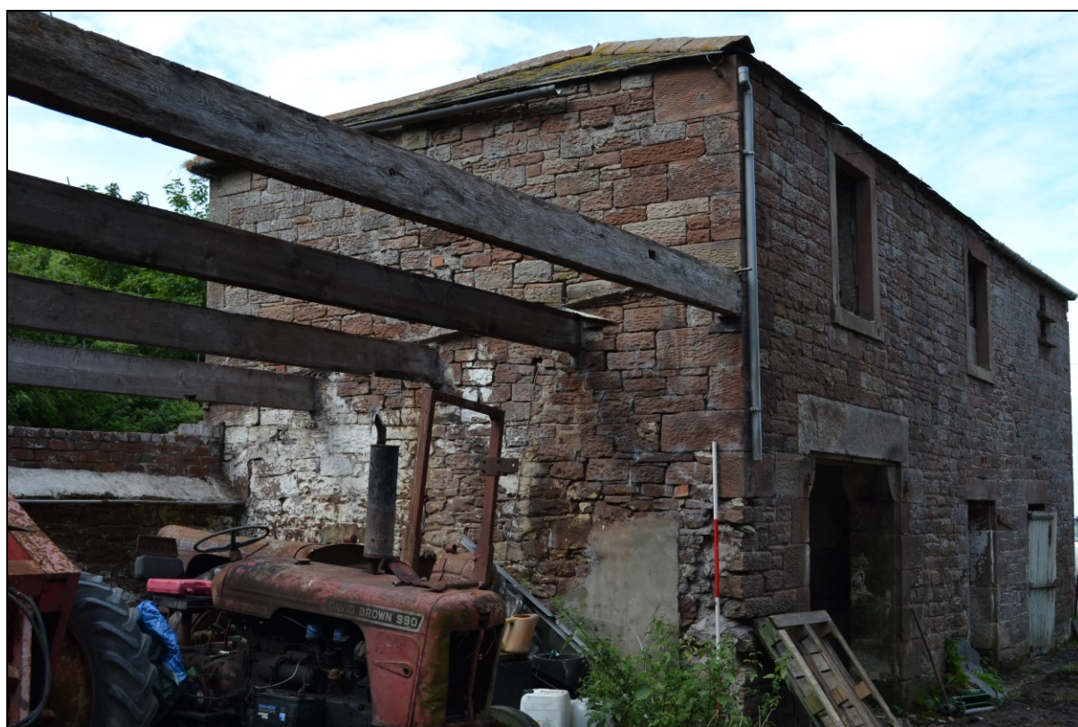
Figure 28. Eastern elevation of stone barn
