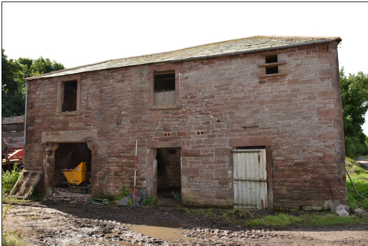
Figure 13. Northern elevation of stone barn
