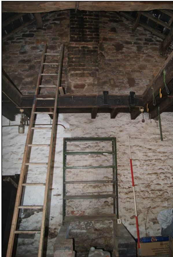
Figure 15. Chimney stack in Building 1
