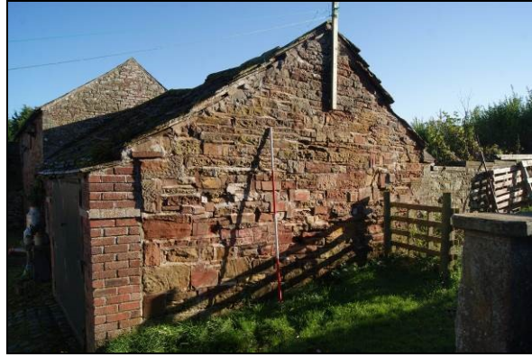
Figure 20. Western elevation, Building 2
