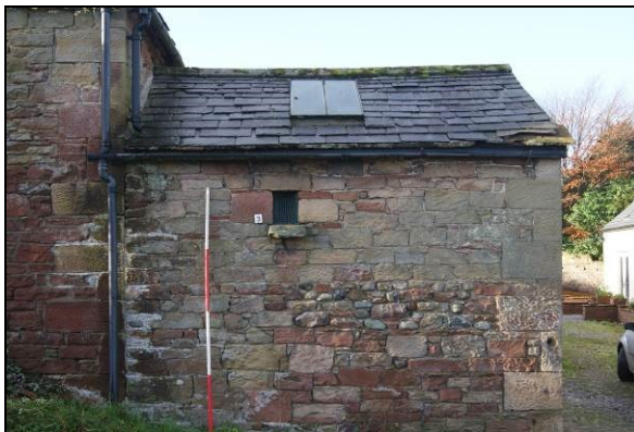
Figure 21. East elevation, Building 3
