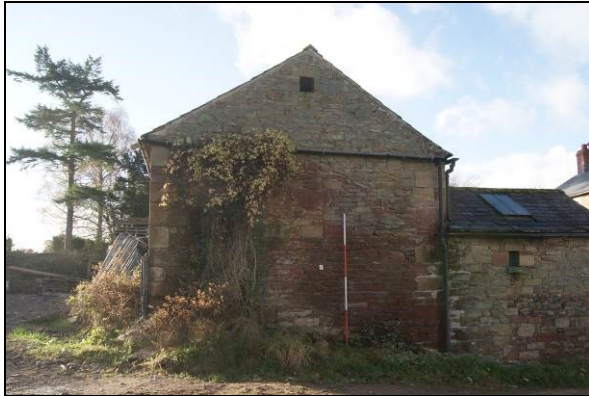
Figure 11. Eastern elevation of Building 1
