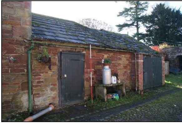
Figure 19. Northern elevation Building 2
