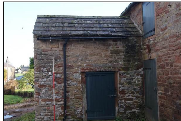
Figure 22. West elevation, Building 3
