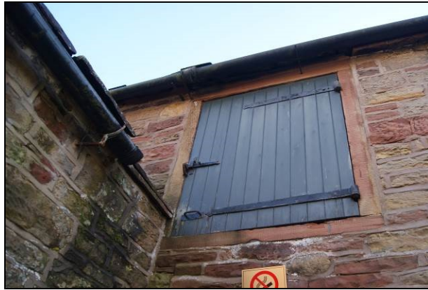
Figure 25. Building 3 butting Building 1
