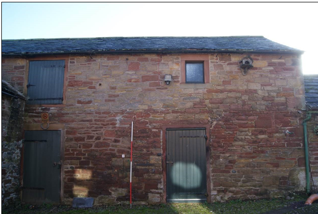
Figure 7. Northern elevation Building 1
