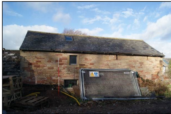
Figure 12. Southern elevation, Building 1
