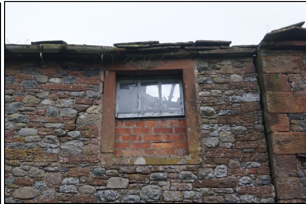
Figure 13. Window (2) within annex
