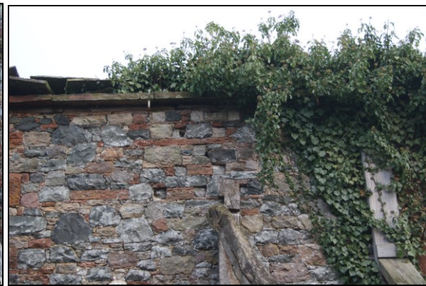
Figure 15. Air vents (6), Room 2
