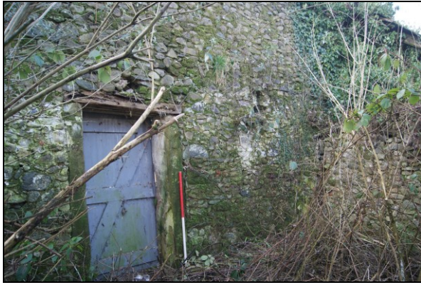
Figure 6. Interior of Room 1
