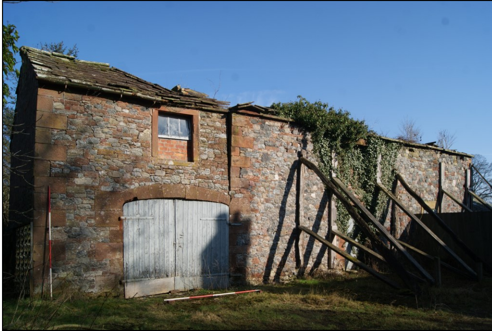
Figure 11. South elevation of the stone barn
