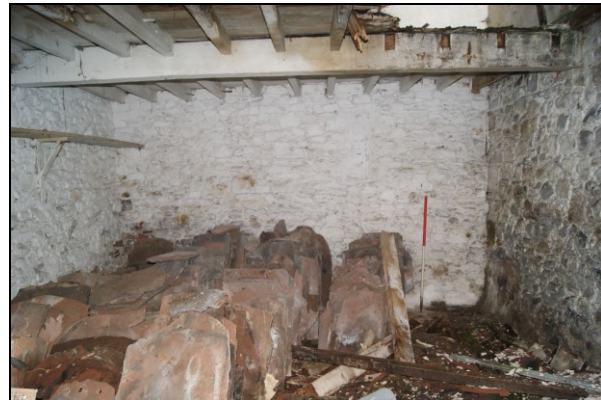
Figure 9. Room 3, lower floor
