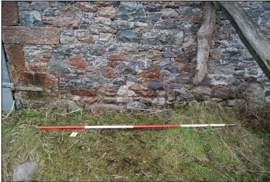
Figure 33. Rounded boulders that may have formed an earlier foundation
