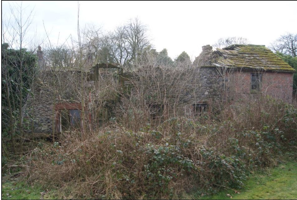
Figure 20. North elevation of barn
