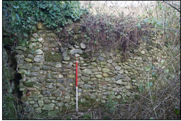
Figure 7. Partition wall on west side of Room 1
