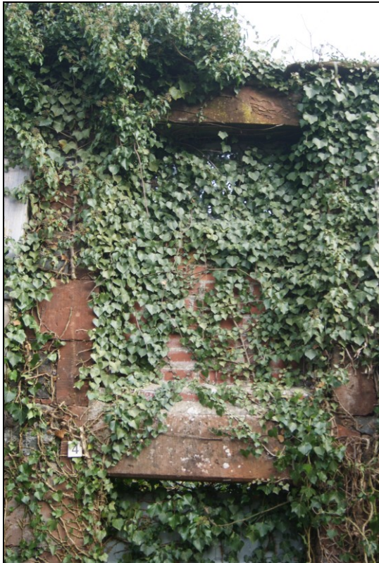
Figure 16. Window (4), above Room 2
