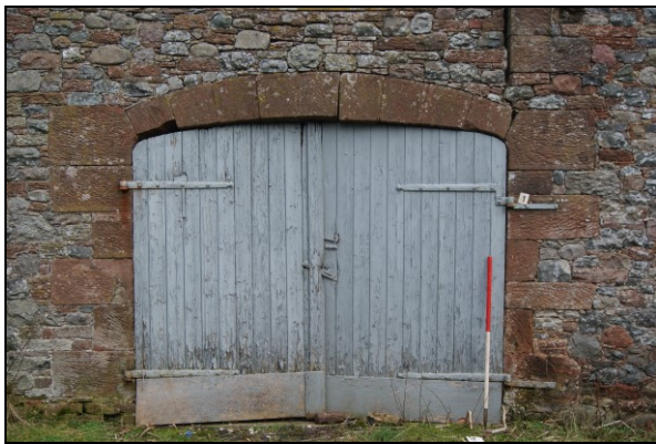
Figure 12. Cart door (1) to annex
