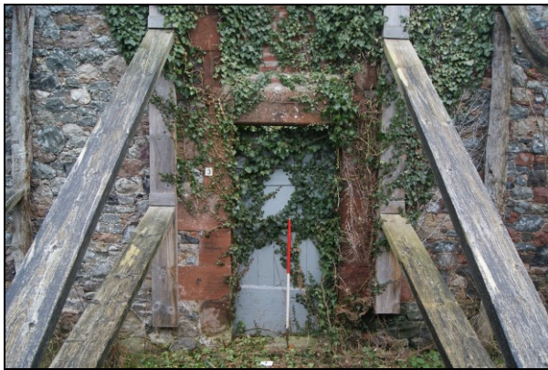
Figure 14. Doorway (3) into Room 2
