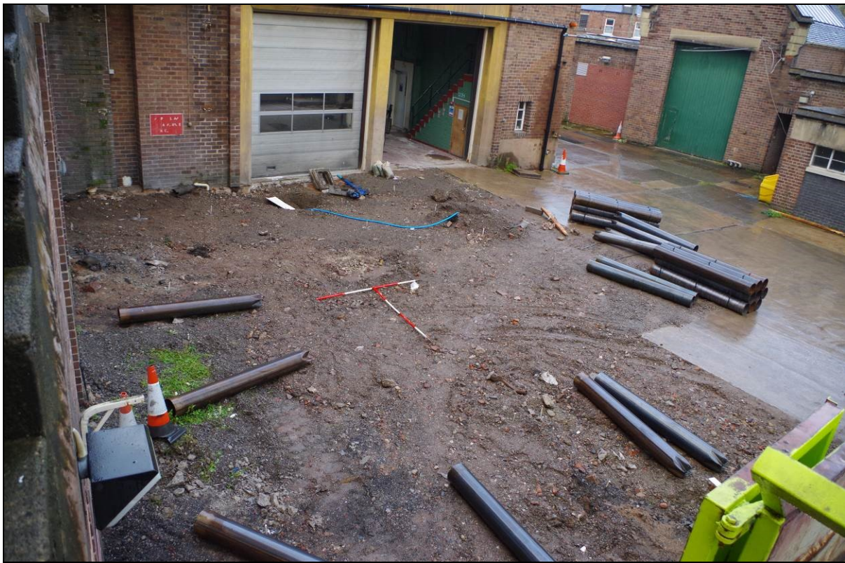
Figure 5. Study area prior to excavation
