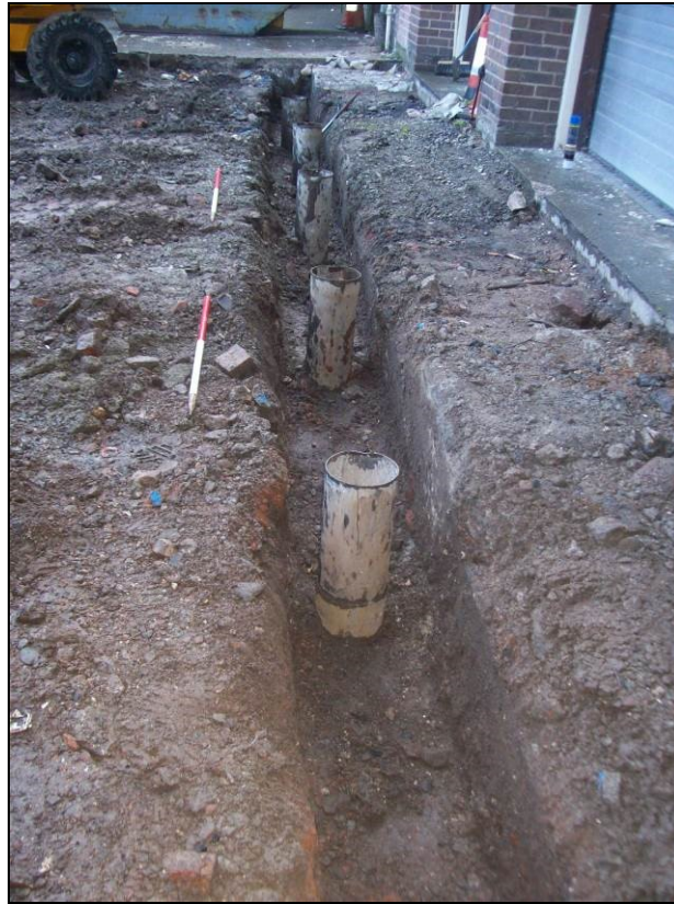
Figure 8. Trench alongside piles
