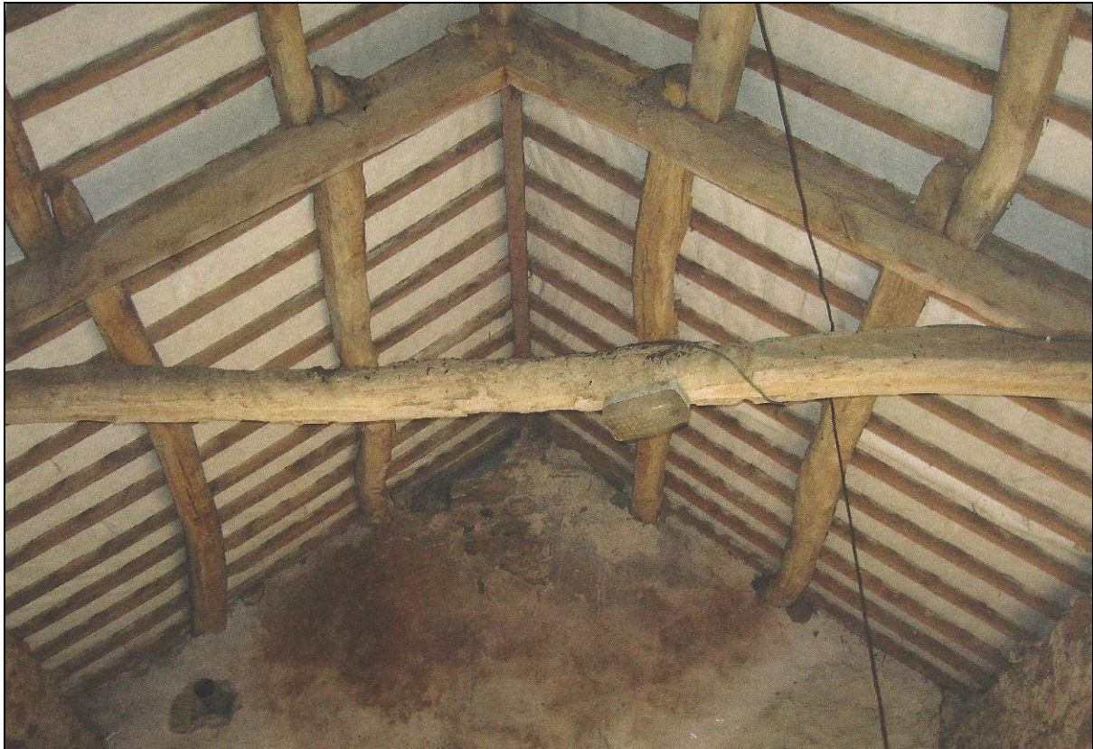
Figure 15. Eastern side of the byre with internal roof timbers
