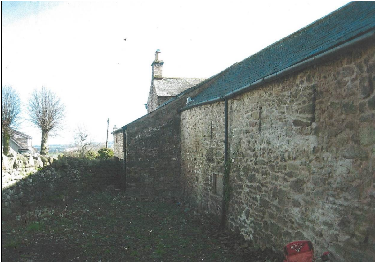
Figure 14. Northern side of the former byre
