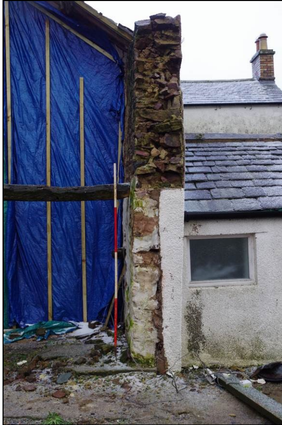
Figure 19. Southern wall of byre
