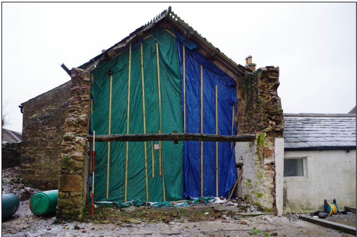
Figure 17. Gable end of former byre
