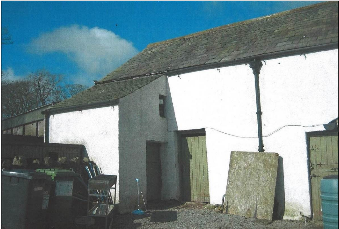
Figure 12. Southern side of the former byre
