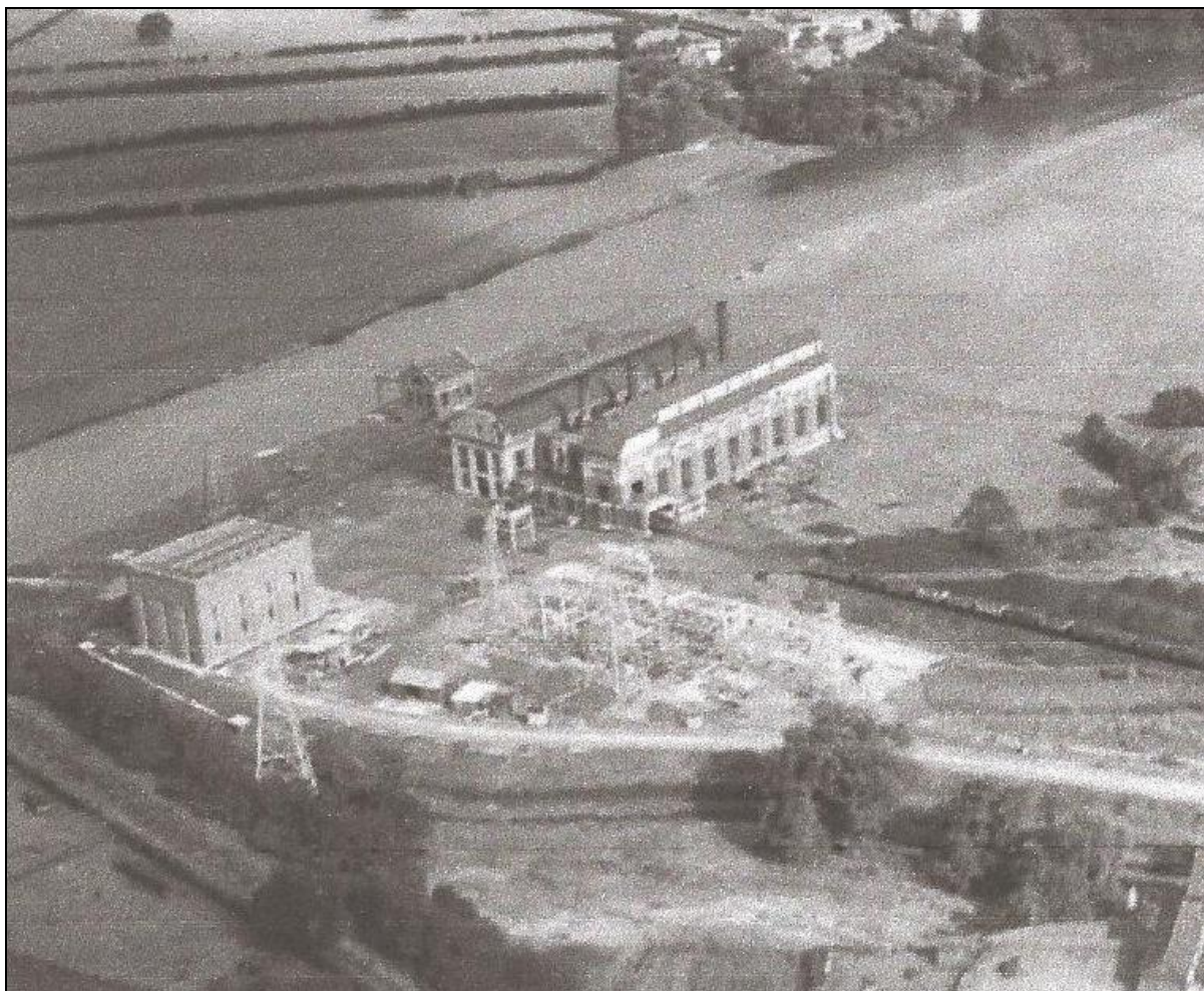
Figure 4. The power station under construction, 1932 courtesy:
