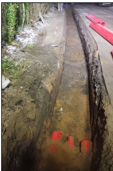
Figure 12. Start of trench
