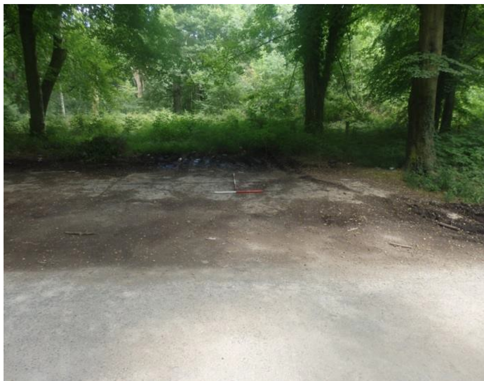
Fig. 6. Hardstanding of the vehicle park.
