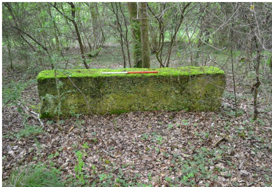
Fig. 7 Concrete block used to support each end of the railway carriage accommodation huts.
