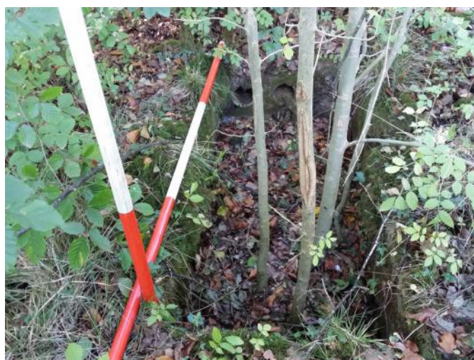
Fig. 17 Large drain with two ceramic pipes entering it from the huts adjacent to the Grand Avenue at SU 2110068203.
