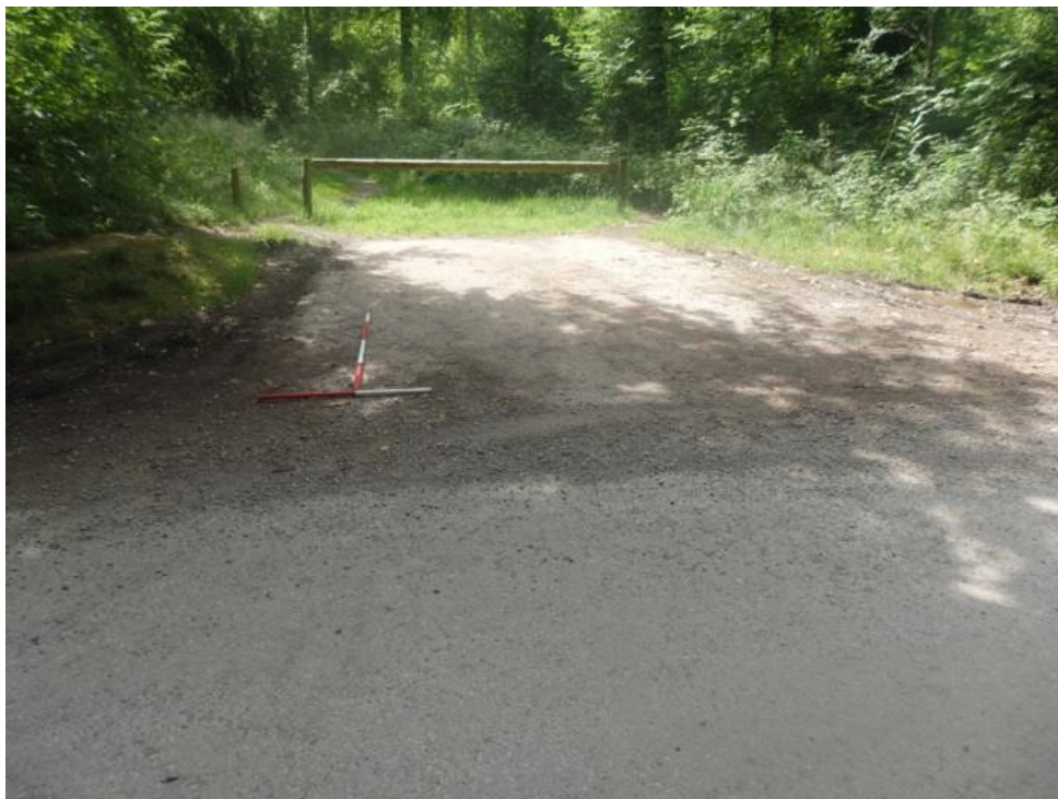
Fig. 5 Entrance to the inner circular road from the Grand Avenue
