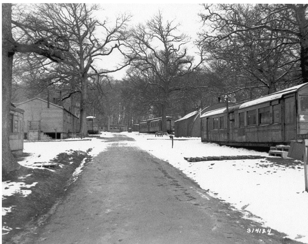
Fig. 10 Contemporary photographs show these huts supported by the concrete blocks and with steps leading to the entranceways. Copyright US National Archives (public domain).
