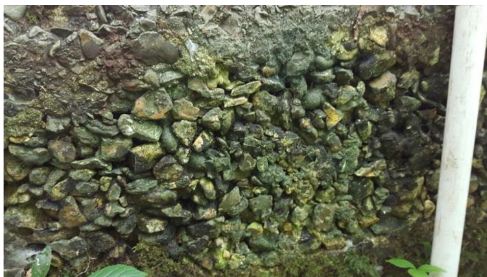
Fig. 8 High ratio of aggregate to cement mix of concrete support blocks.
