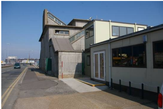
Figure 15. West end of south elevation looking north.
