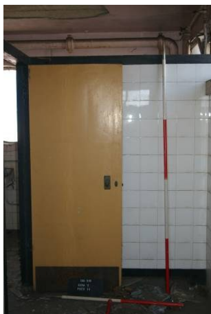
Figure 54. Lobby to room 12 looking west.
