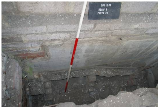
Figure 44. Exposed structure below bridge entrance looking west.
