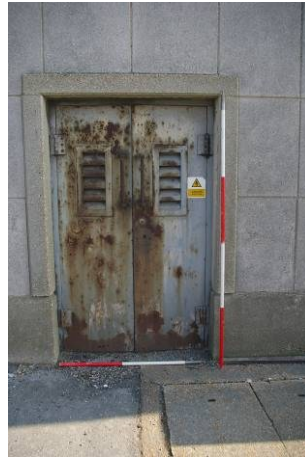
Figure 11. Door to room 1 looking east.
