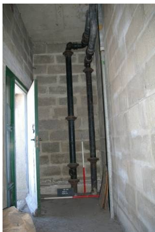
Figure 36. Room 5 looking east.
