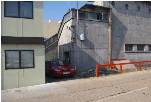
Figure 16. East end of the south elevation looking north-west.
