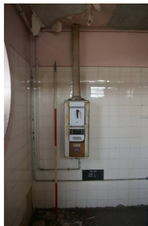
Figure 53. Incinerator on north wall of room 11 looking north.
