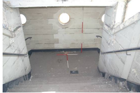
Figure 45. Room 8 looking east.
