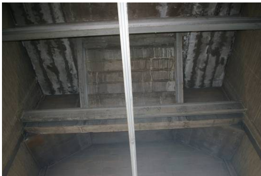
Figure 30. Room 2 ceiling looking east.
