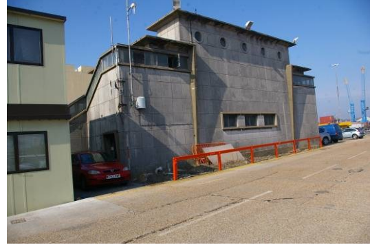
Figure 17. East elevation looking north-west.
