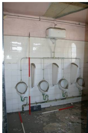
Figure 57. Urinals against the south wall of room 12 looking south-west.
