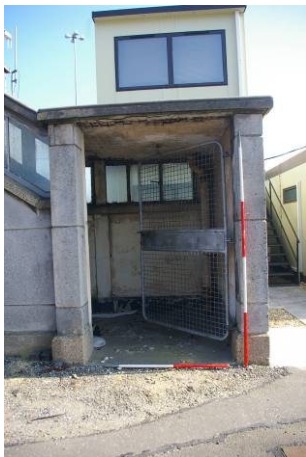
Figure 10. Gate to stairwell room 6 looking east.
