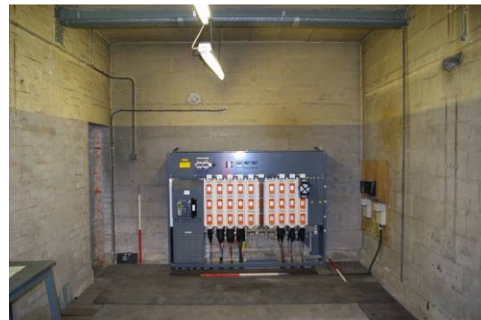
Figure 19. Room 1 looking east.
