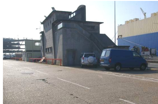
Figure 18. North and east elevations looking south-west.
