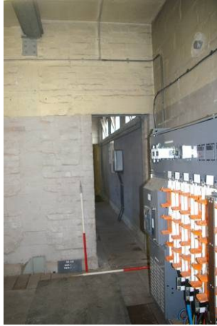
Figure 21. Doorway from room 1 to room 2 looking north.
