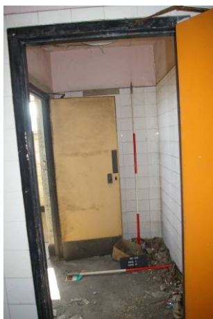
Figure 49. Lobby to room 11 looking south.
