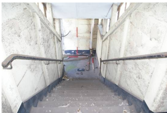
Figure 48. Lower flight of room 10 looking north.
