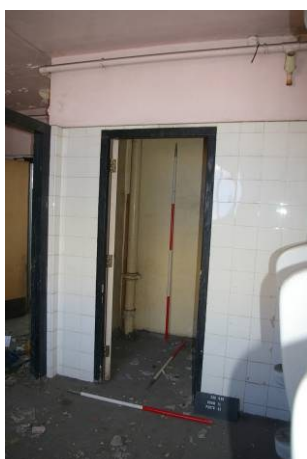
Figure 56. Room 12 looking east.
