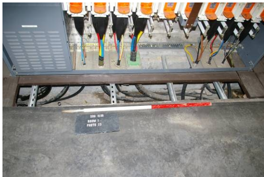
Figure 22. Cable trench against east wall of room 1 looking east.
