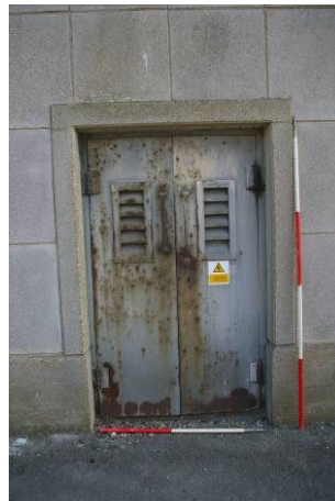
Figure 13. Door to room 3 looking east.
