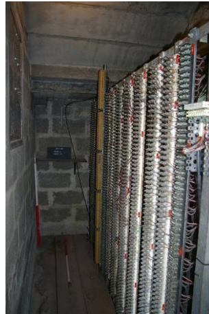
Figure 33. Room 4 looking west.
