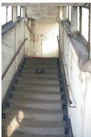
Figure 38. Lower flight of room 6 looking north.
