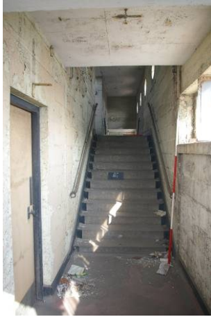
Figure 42. Room 7 looking north.
