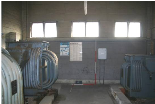
Figure 23. Room 2 looking east.
