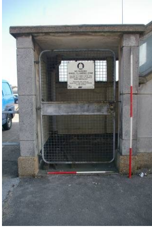
Figure 14. Gate to stairwell room 10 looking east.
