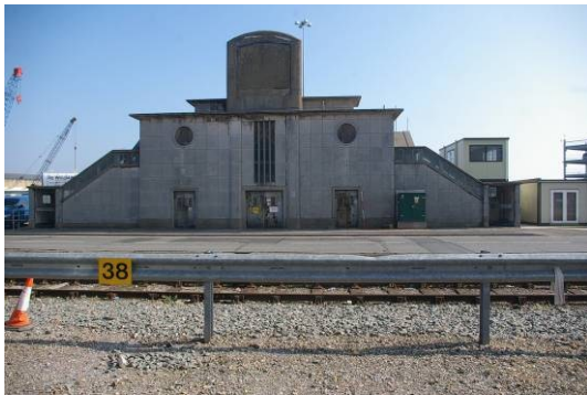
Figure 9. West elevation looking east.
