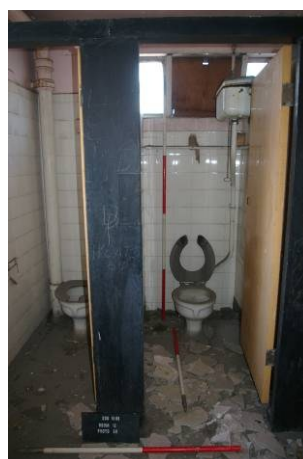
Figure 58. Toilet cubicles against the north wall of room 12 looking north.
