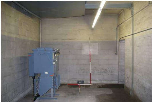
Figure 31. Room 3 looking east.
