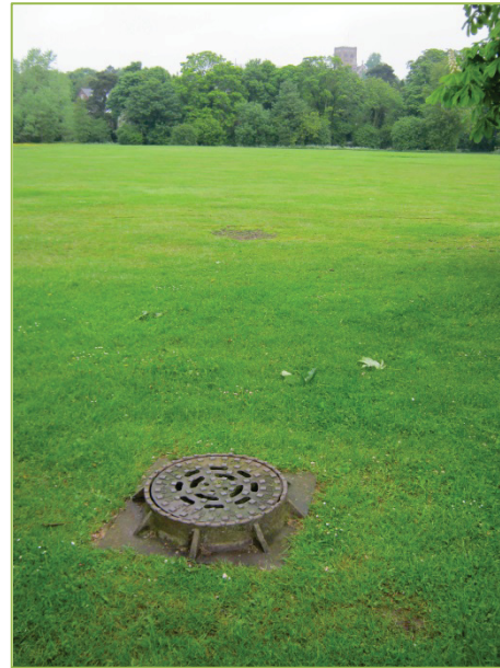
Manhole 0602, Looking North-east along the line of the proposed sewer upgrade.
