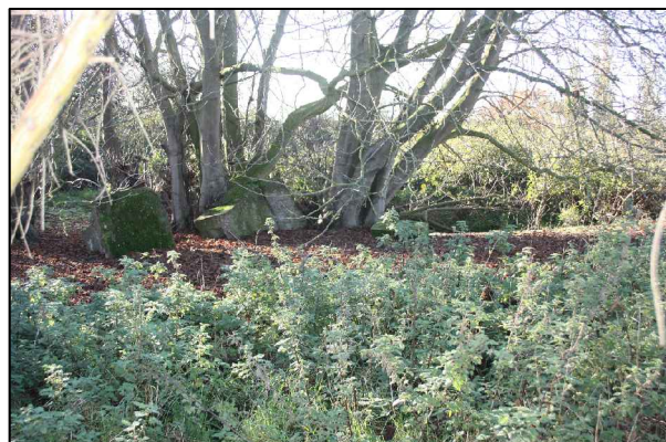
DP10- Concrete Blocks, Possible Former Entrance - Looking West
