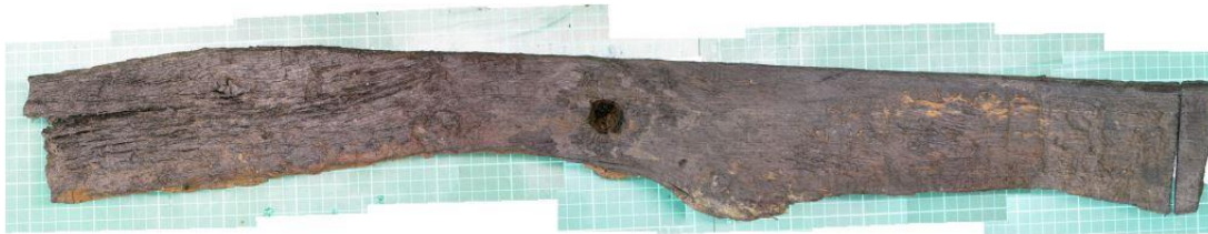
Figure 23 Photograph of timber 20
