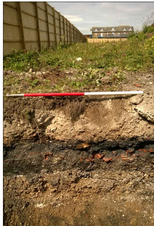
DP24 - Sample Section 6b - View NW
