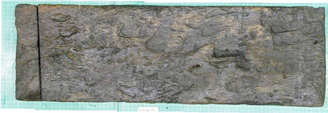
Figure 29 Photograph of timber 22
