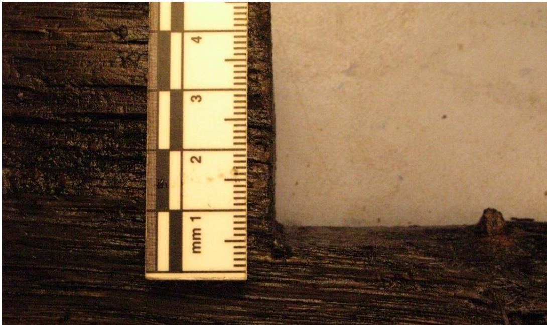
Figure 68 Photograph showing saw overcut and iron fitting on timber 74
