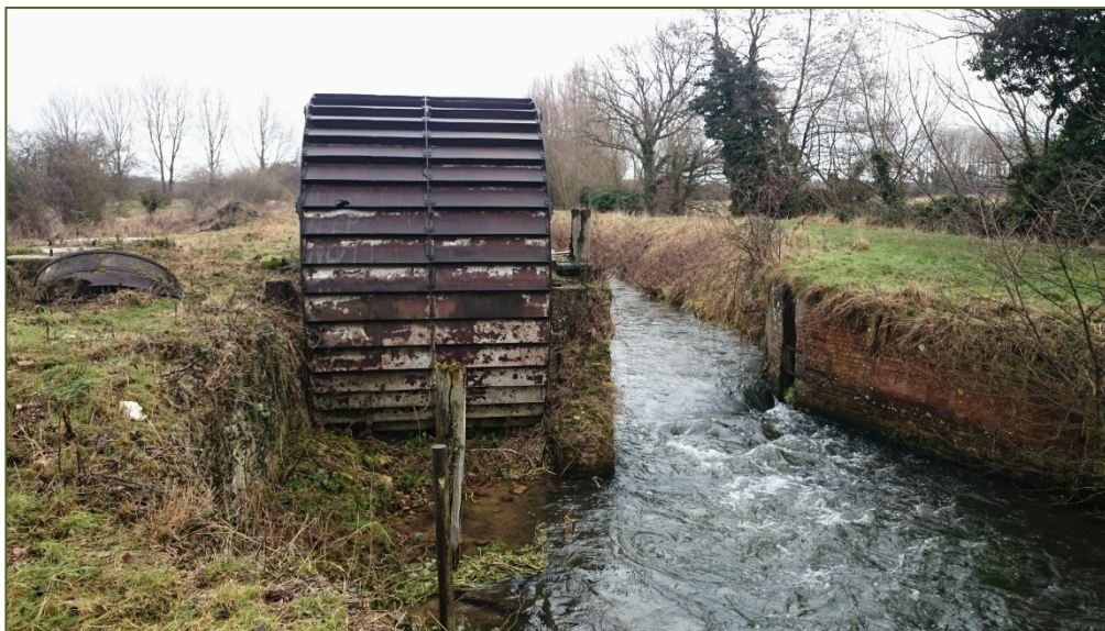
Low-breast Water Wheel, Facing north-east from the south-west.
