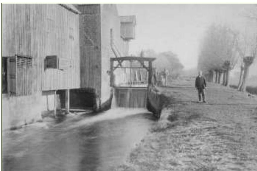
Photograph dated c.1890, Facing north-east from the south-west, showing stanch gate.
