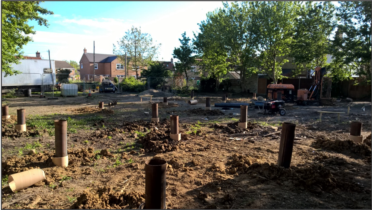
Photo 1: View of northern area of site after pile installation.
