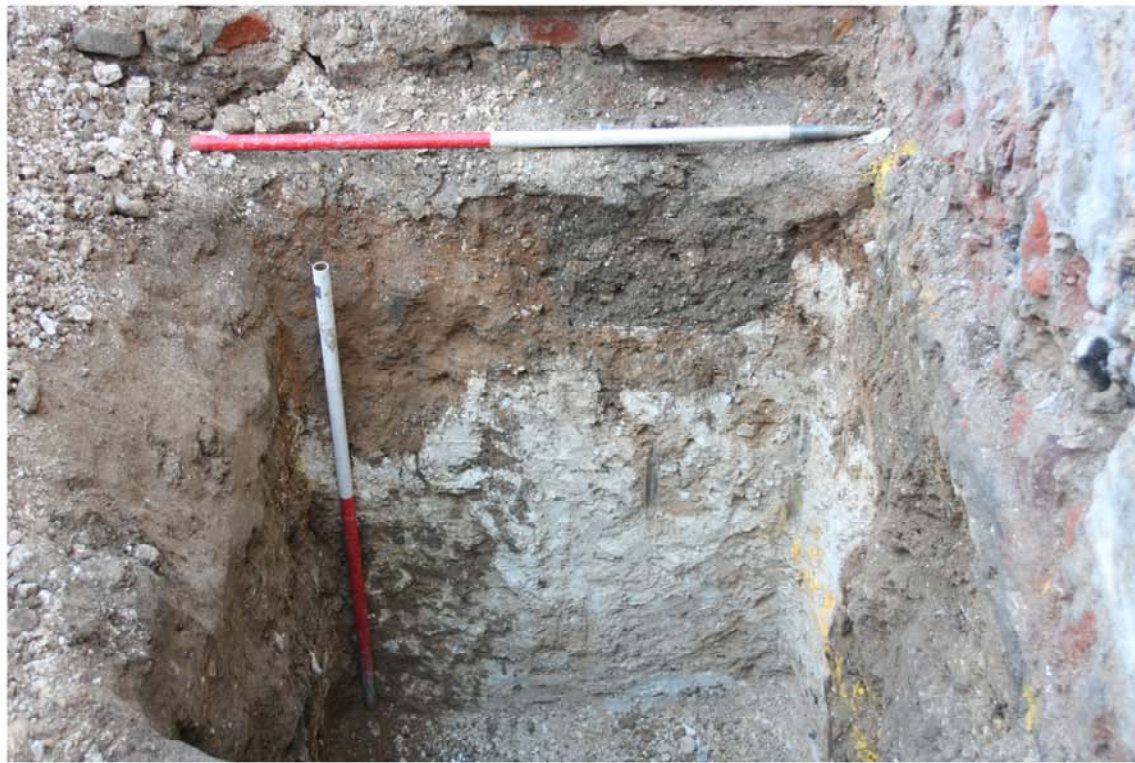
DP 1 - SITE SECTION 1 - VIEW W
