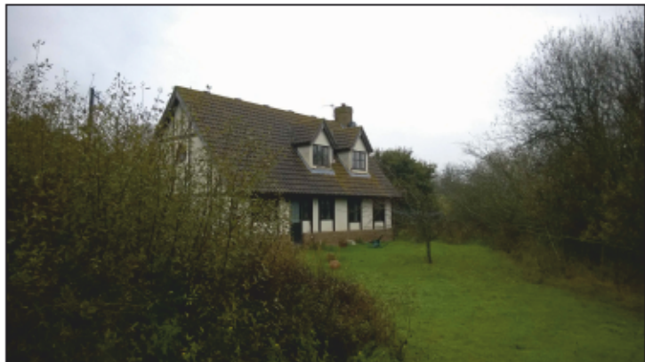
DP7- House in NW Area. View N
