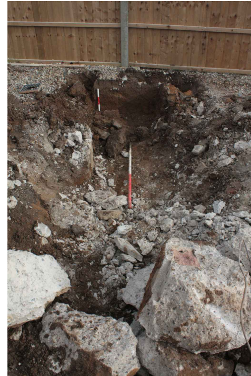
DP:02 - REMOVAL OF CONCRETE PAD
