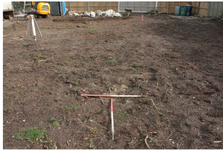
DP:01 - SITE PRIOR TO GROUNDWORKS
