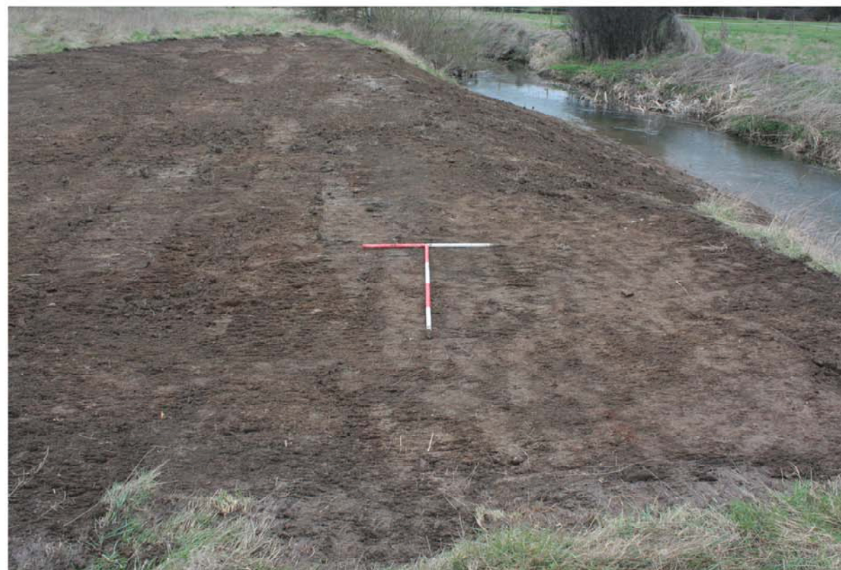
DP 2 - Ground Reduction for Berm - View W
