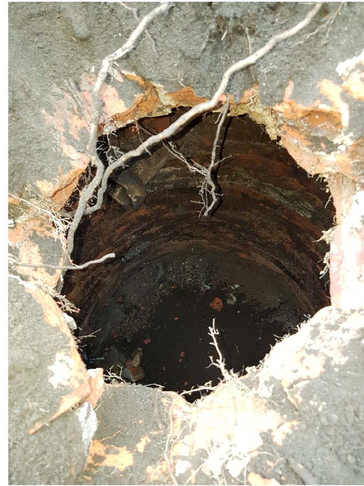
DP 6 - WELL 1004 & CAP - VIEW SW
