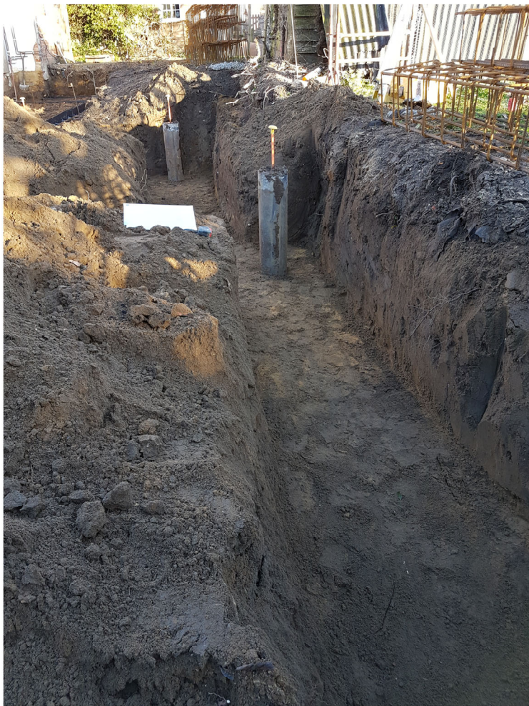
DP 4 - N EXTENT OF FOOTINGS - VIEW N
