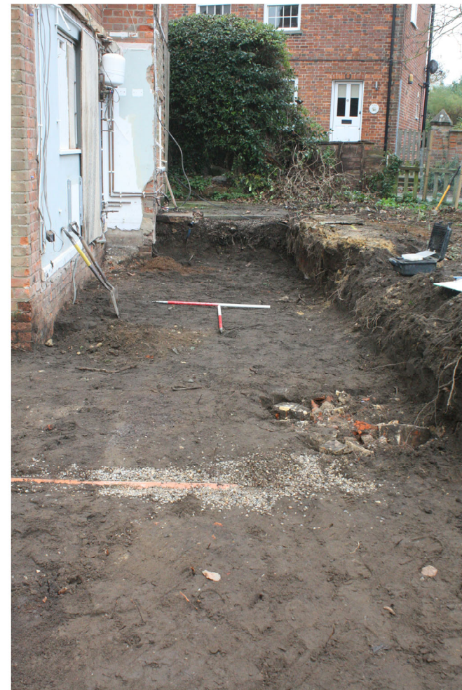
DP 2 - NE SITE, 1001 EXPOSED - VIEW NE
