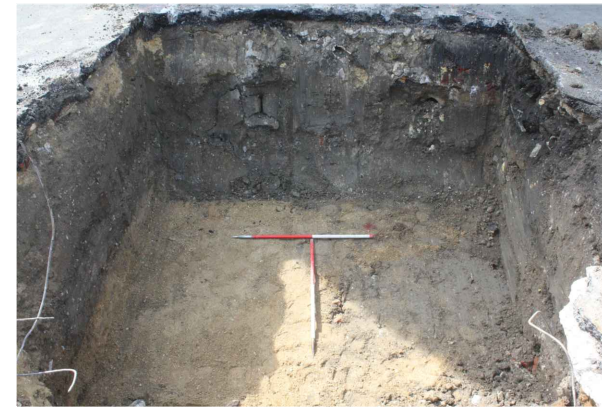
DP 2 - TEST PIT 1
