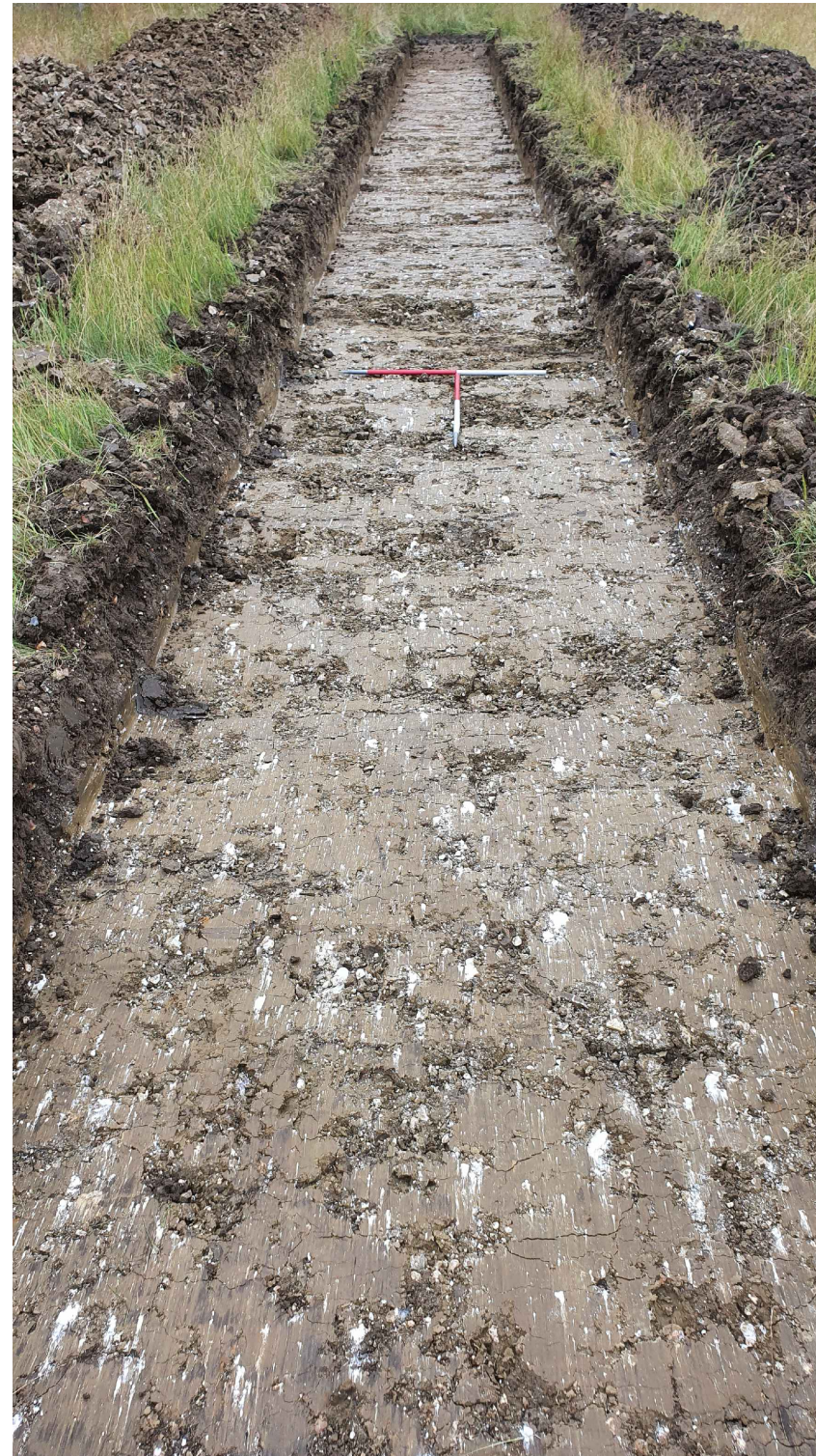
DP09 - TRENCH 4 - VIEW NW
