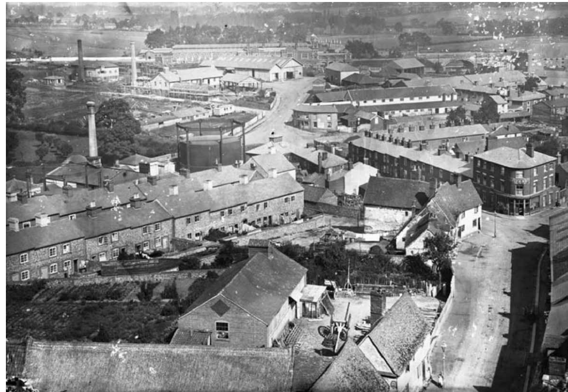
Photograph dated 1871 showing the original retort house from 1834. View NE
