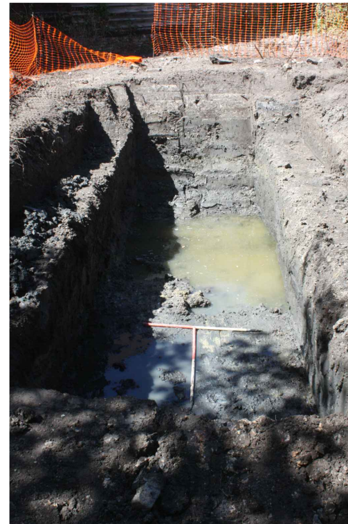
DP 2 - TRENCH SHOT, VIEW NW
