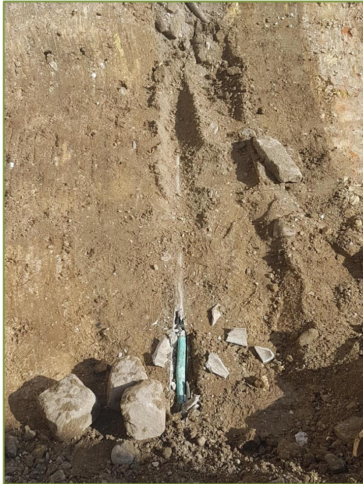
DP20; Test Pit 5 – Service pipe showing service run and level that excavation ceased.
