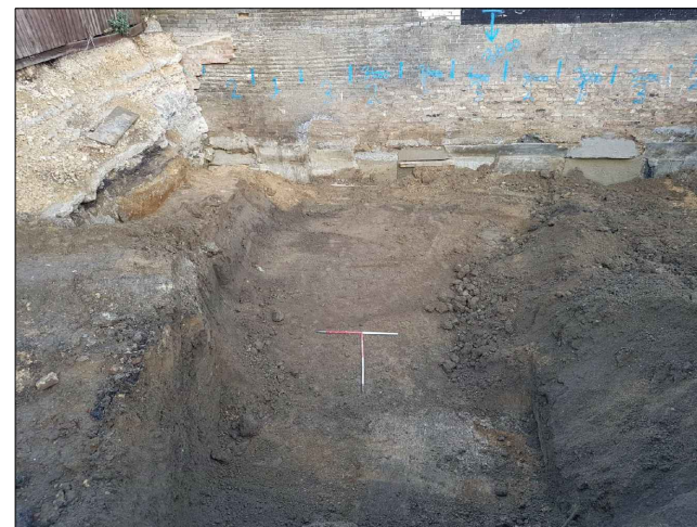
DP:3 - EXCAVATION AREA S END, VIEW E
