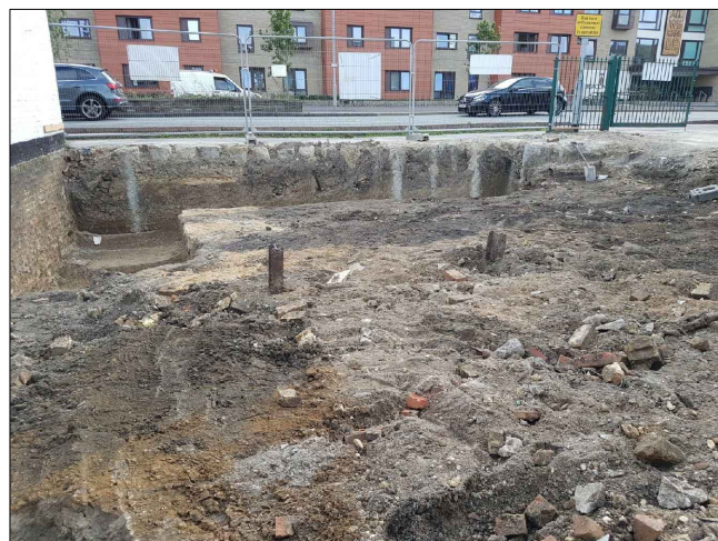
DP: 6 - SITE VIEW S
