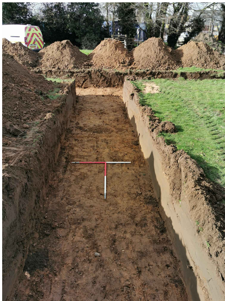
DP8 - TRENCH 4 - VIEW NW
