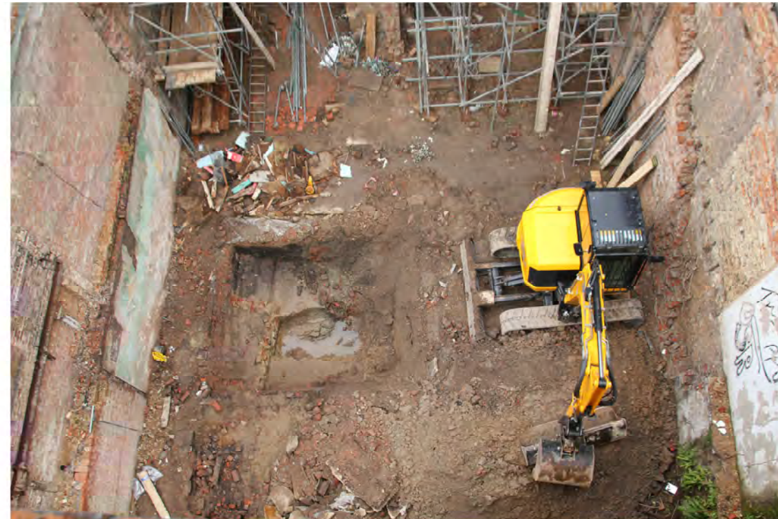
OVERALL SITE SHOT DURING TP1 EXCAVATION
