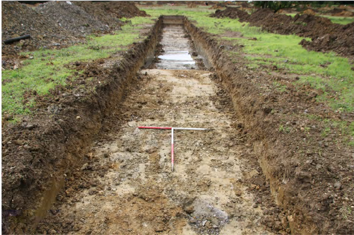
DP37 - TRIAL TRENCH 15 - CHANNEL 1049 - VIEW SE
