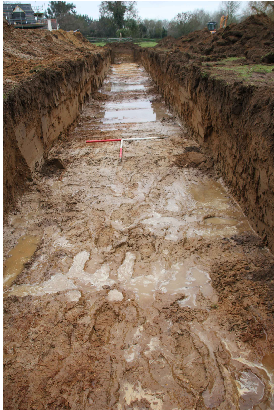
DP4 - TRENCH 2 - VIEW NW
