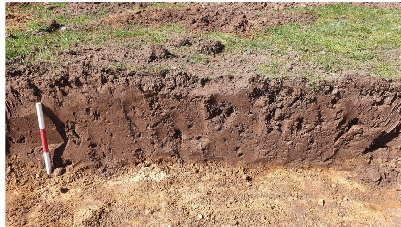
DP3 - SAMPLE SECTION 2 - VIEW W
