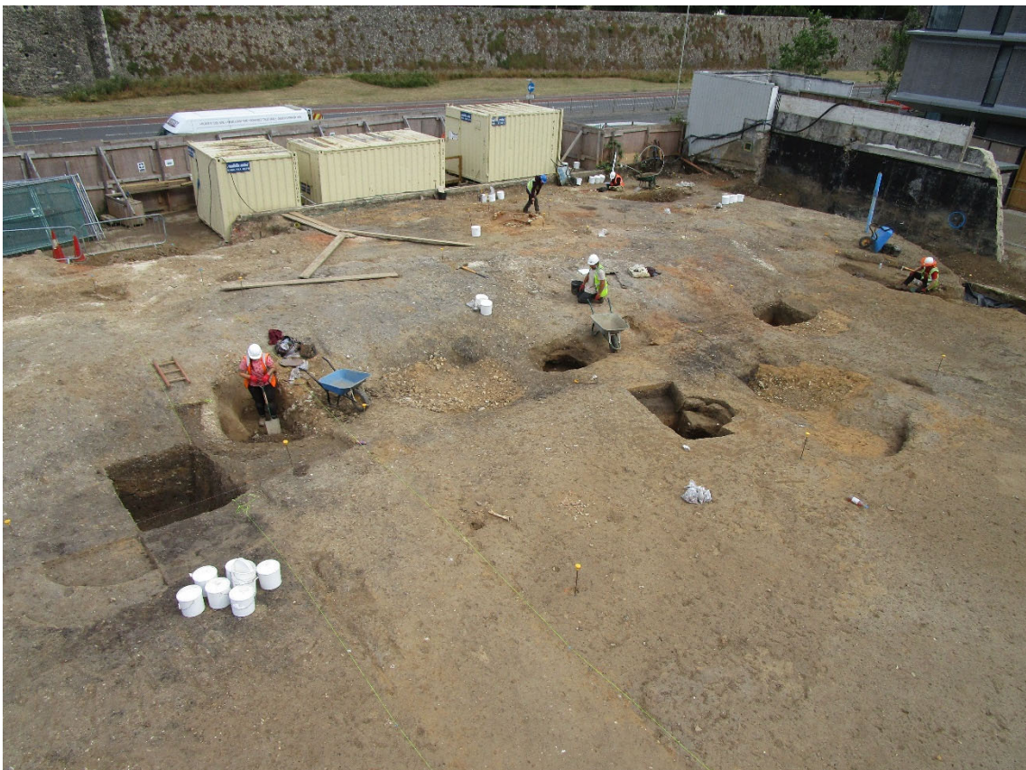
Photo 30. G27 pits during hand excavation, looking north (no scale)
