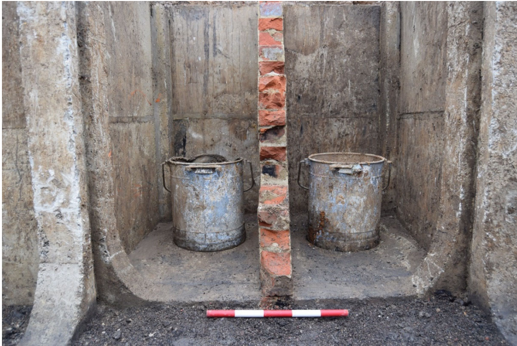
Photo 53. G36 concrete-lined air raid shelter, detail of latrine cubicle with in situ galvanised steel buckets (SF 1 and SF2), looking southeast (scale 0.5m)
