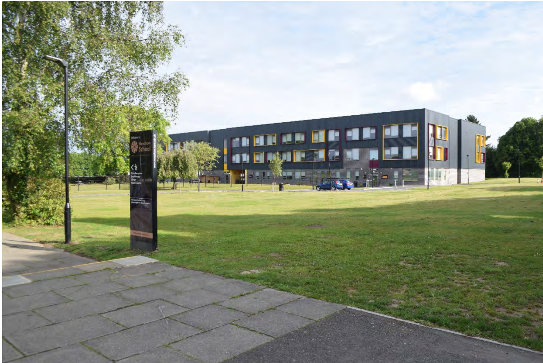
Plate 1. Pre-excitation, Area A east side, looking north-west
