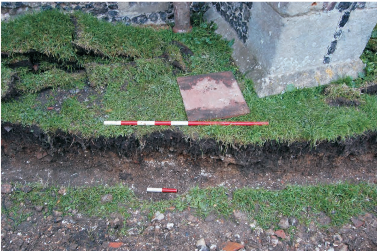
Plate 11: Southern pipe trench, looking north-east (Scale 1m and 0.5m)
