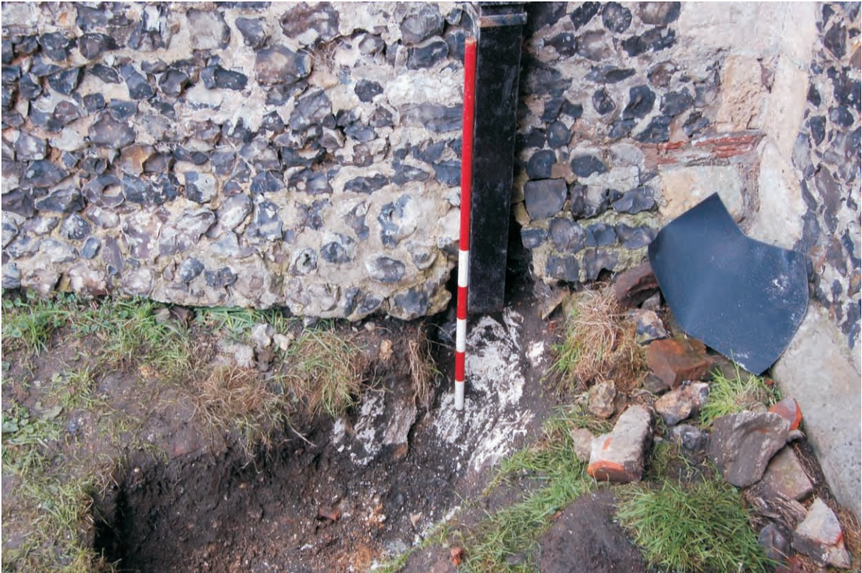
Plate 9: South transept downpipe (east), looking north-west (Scale 1m)
