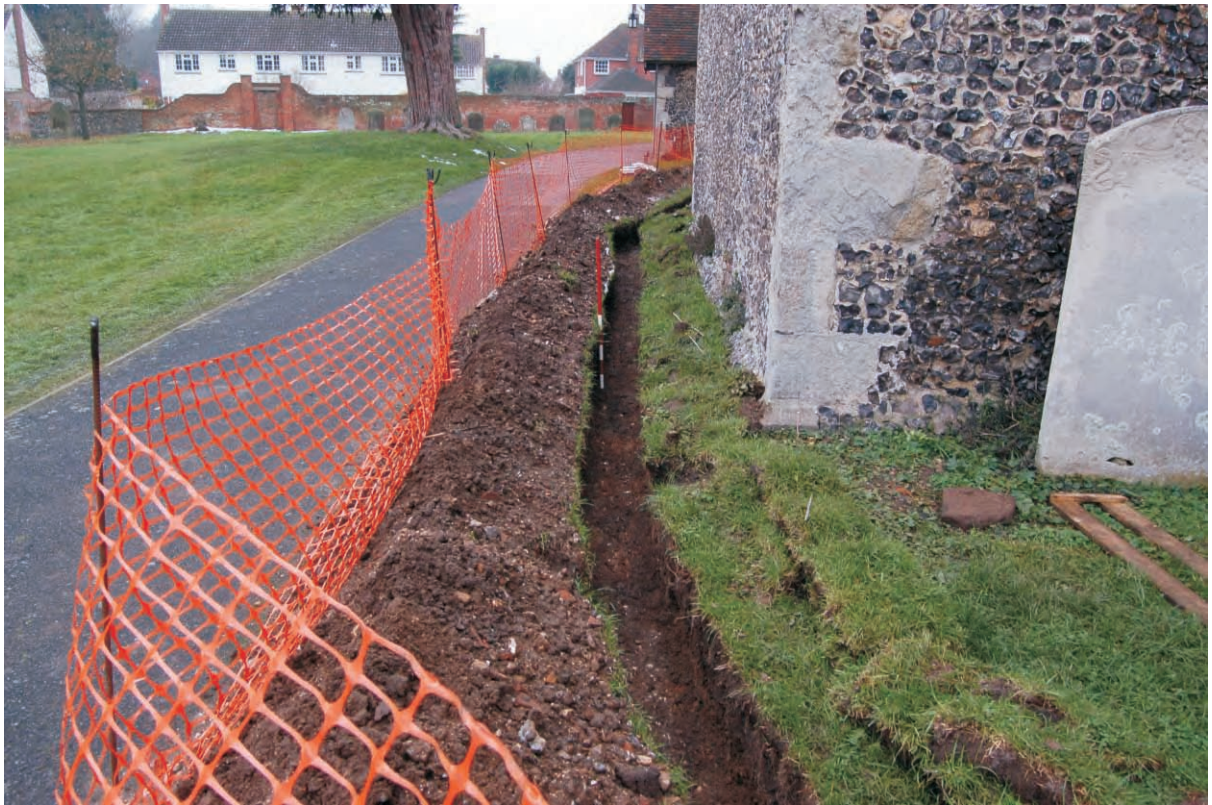
Plate 10: South transept and southern pipe trench, looking west (Scale 1m)
