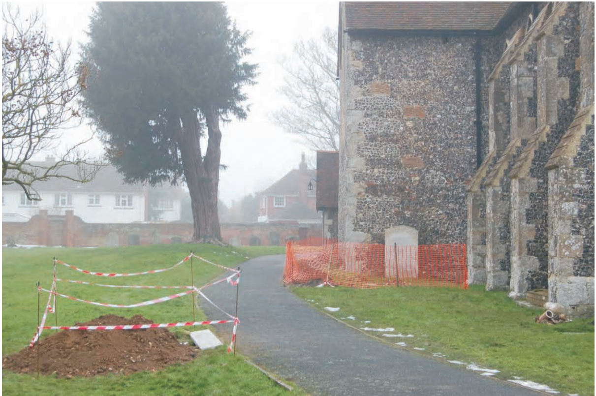
Plate 1: Works underway at Chartham Church, winter 2010-11
