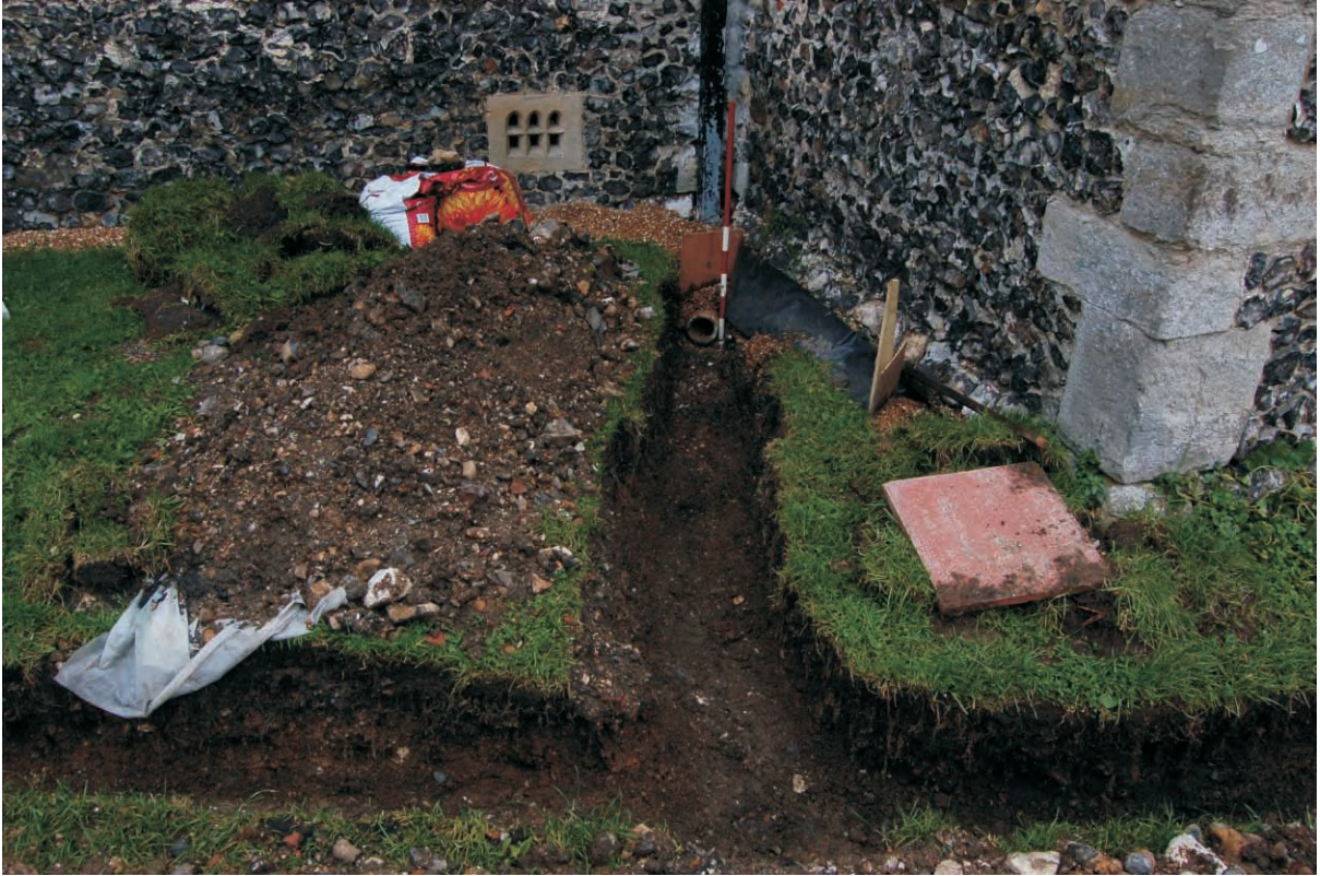
Plate 8: South transept downpipe (west), looking north-east (Scale 1m)
