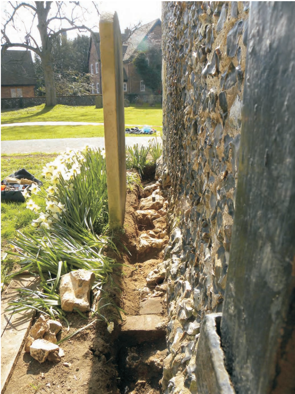
Plate 18: General shot of pea-shingle trench, looking south
