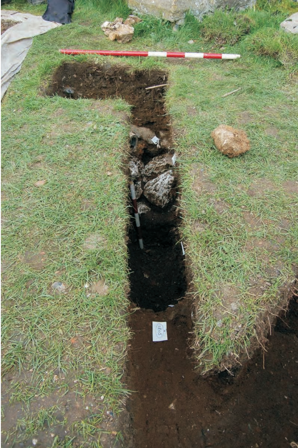
Plate 13: South-eastern pipe trench extension and void, looking north-west (Scale 1m and 0.5m)
