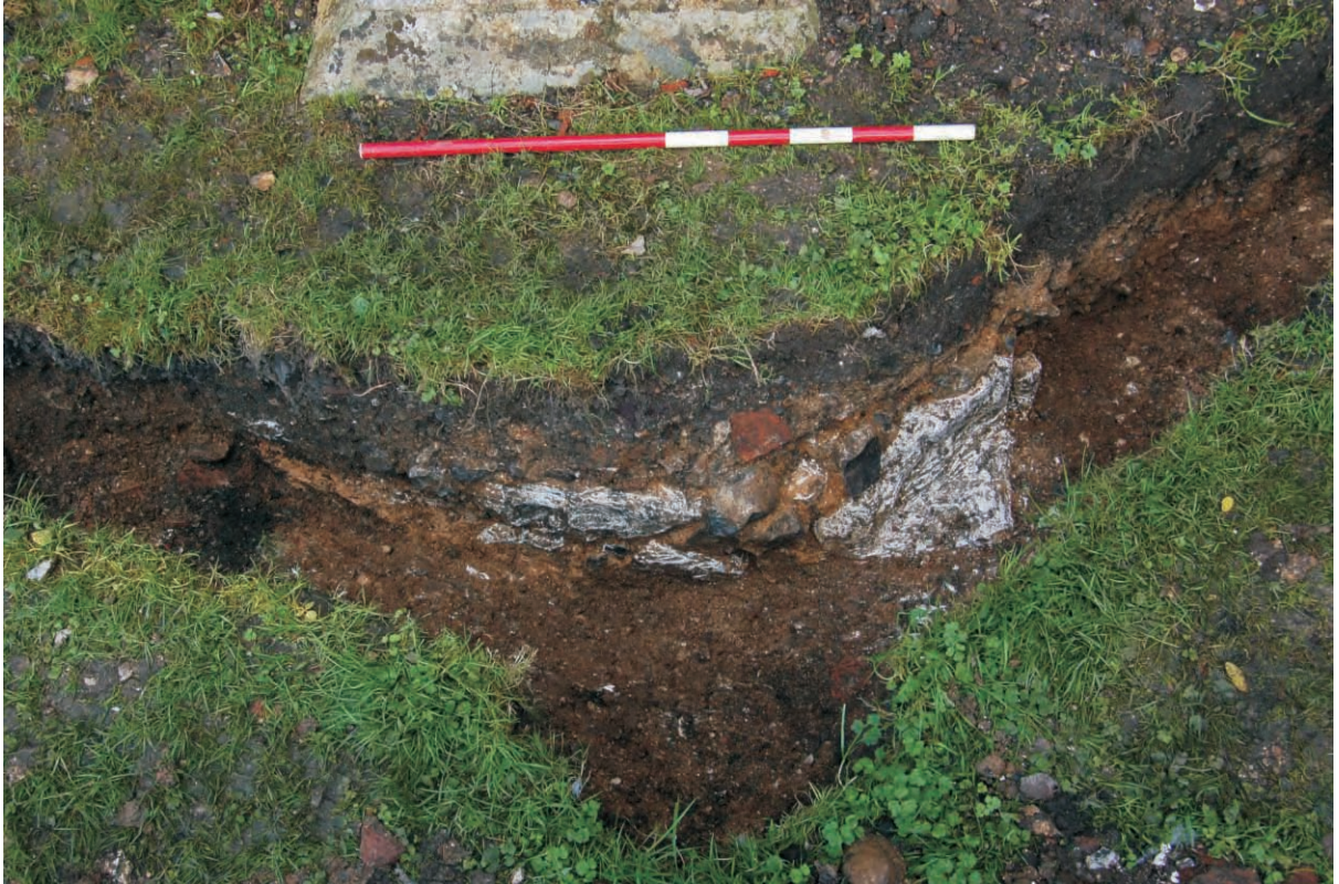
Plate 2: Chancel buttress foundation in the north-east pipe trench, looking south (scale 1m)
