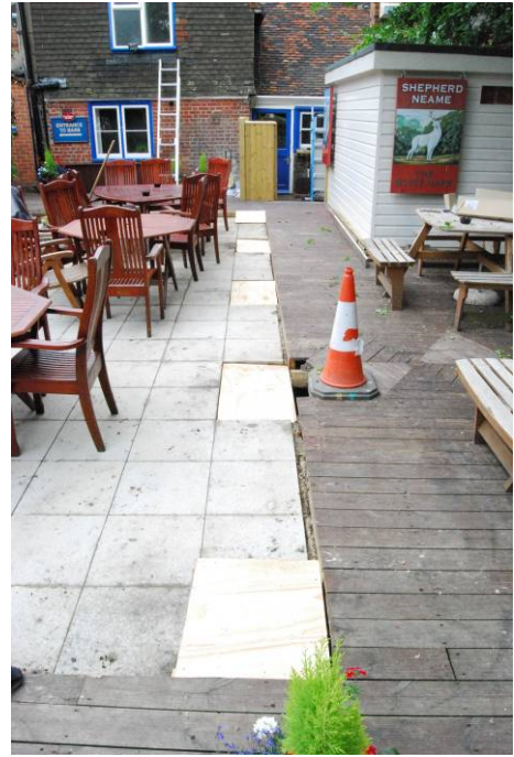
Plate 10. General view of proposed development area after groundworks, looking south-west
