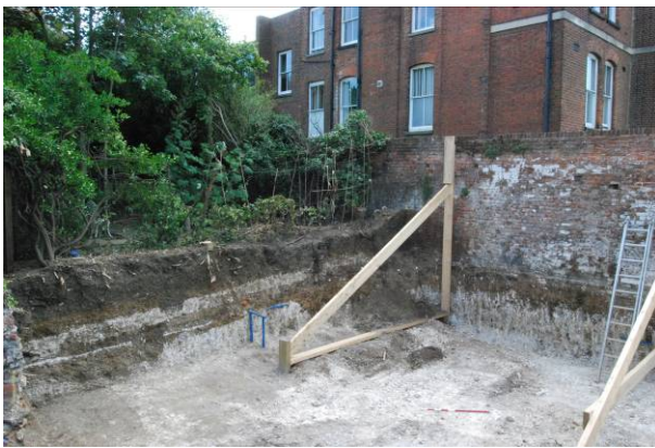
Plate 2. General view of proposed building footprint after groundworks, looking north-east
