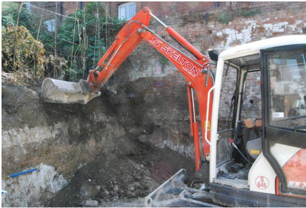
Plate 1. Machine excavation of raised rear garden area, looking north-east
