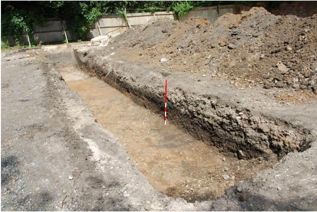
Plate 5 Trench 1 north-west facing section, looking east, scale 1m
