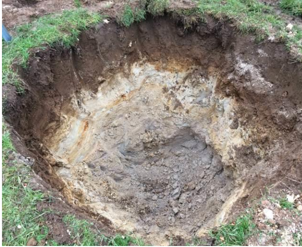
Plate 1: Pit for new treatment plant. No scale
