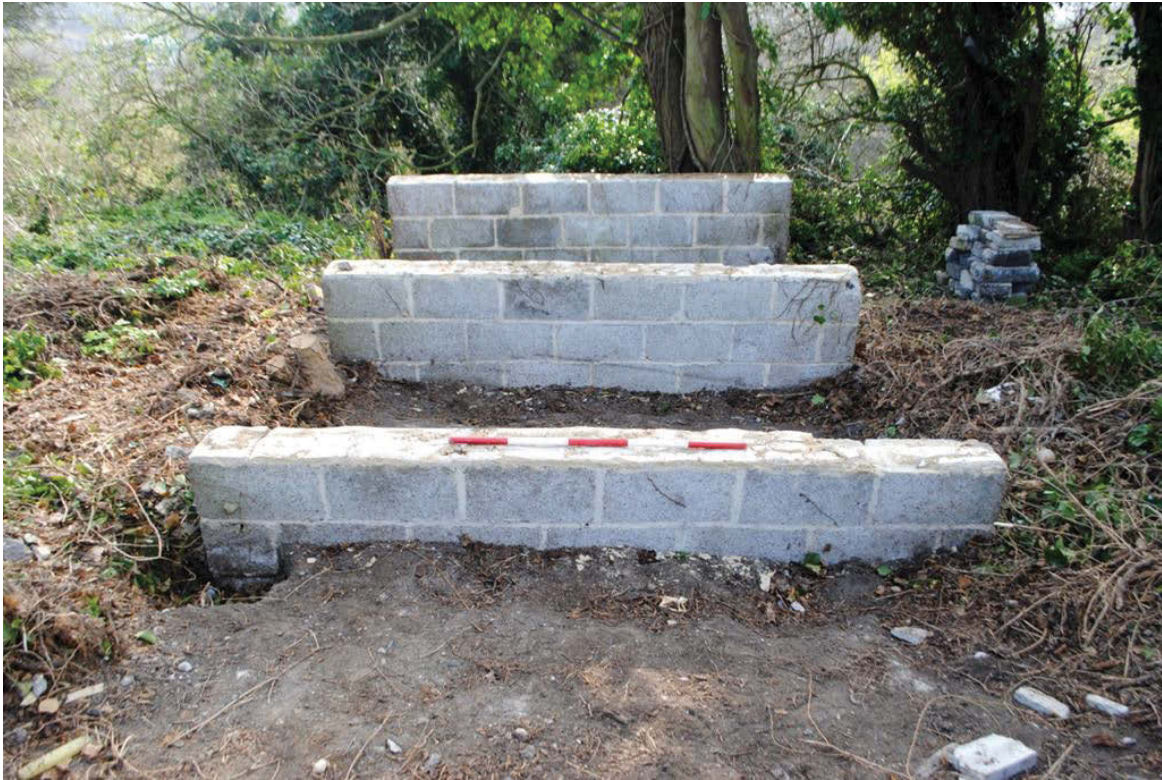
Plate I Foundations of the demolished garage building before excavations began, looking east. Scale, one metre (CAT Film No. 16898, 0132)
