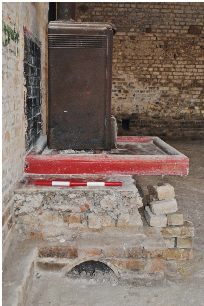
Plate V Room 20, later fireplace over earlier one, looking NW (note vent pipe below earlier hearth). Scale, 50cm (Film 16881/25)
