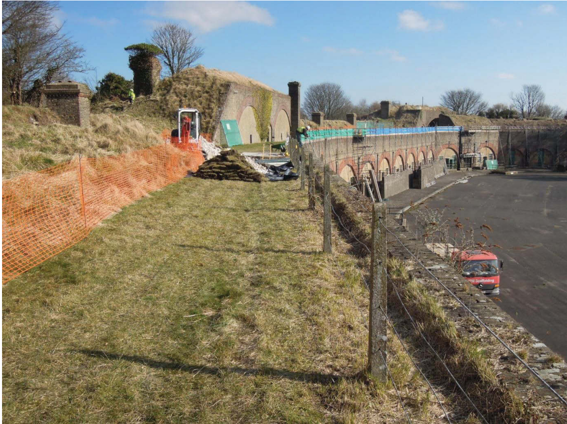
Plate III Trial Pit 2 under excavation, looking east (Film 16863/2667)
