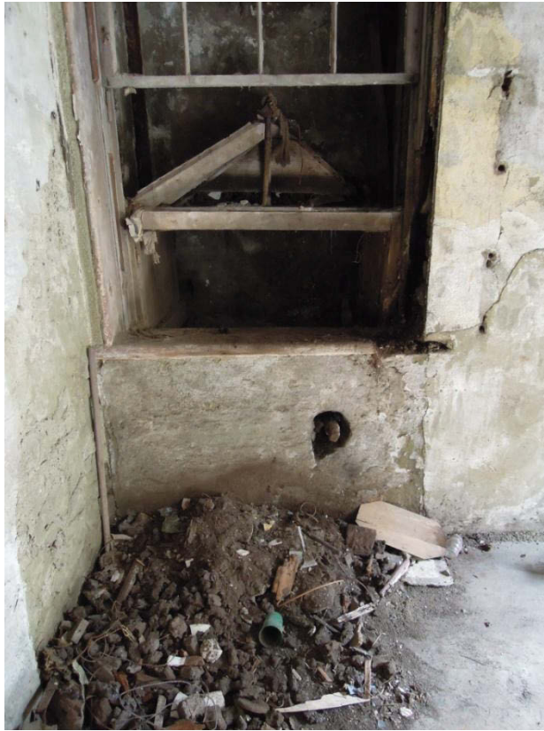
Plate VIII Basement Room 23, shaft for 'dumb waiter' exposed, looking SE (Film 16880/2930)
