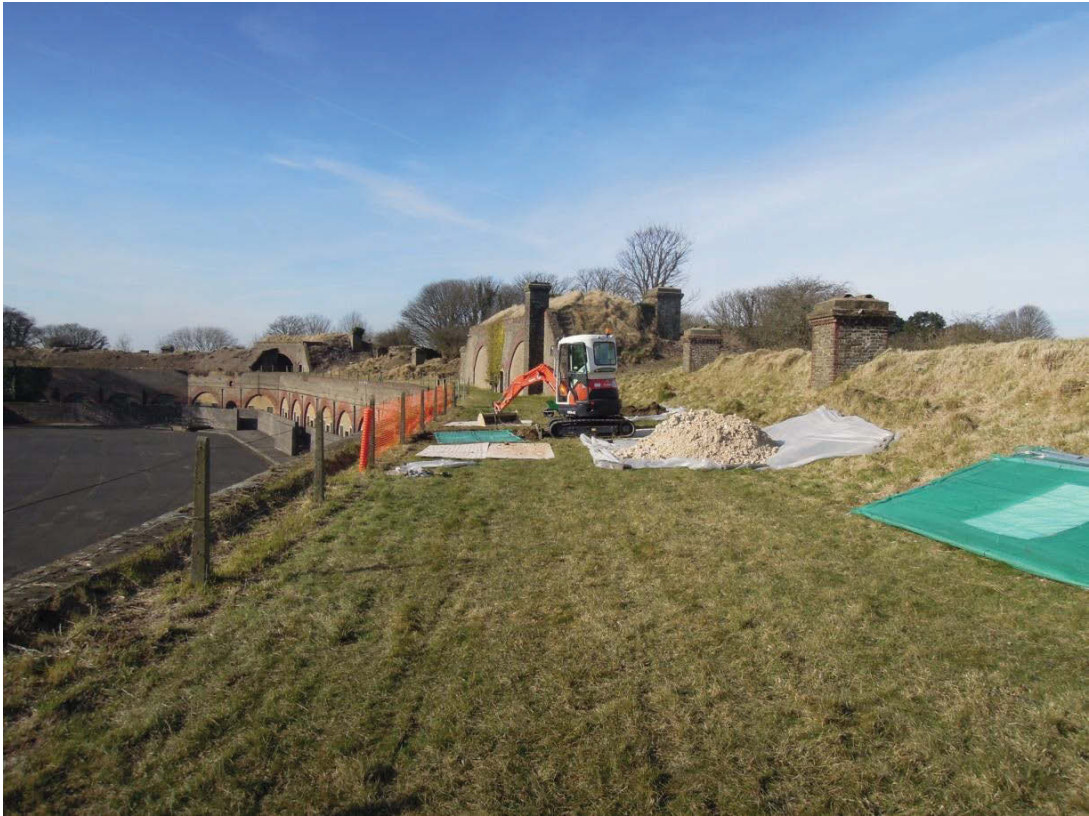
Plate II Trial Pit 1 under excavation, looking north-west (Film 16862/2628)
