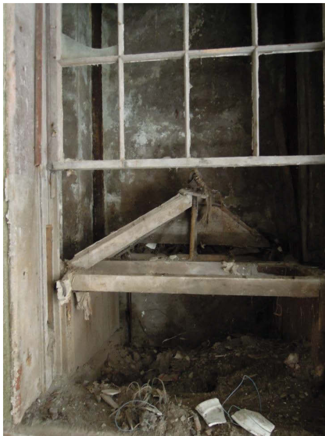
Plate IX Basement Room 23, detail of 'dumb waiter' revealed, looking SE (Film 16880/2924)
