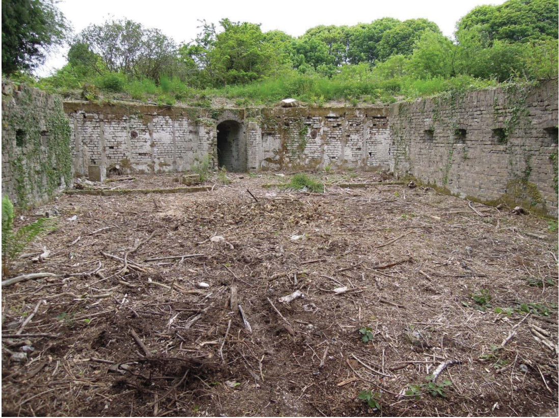
Plate X Barbican structure (Room 50) before clearance, looking north (Film 16893/3157)
