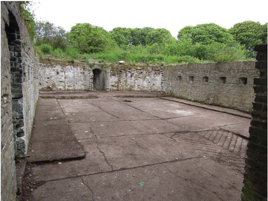
Plate XI Barbican structure (Room 50) after clearance, looking north (Film 16894/3208)
