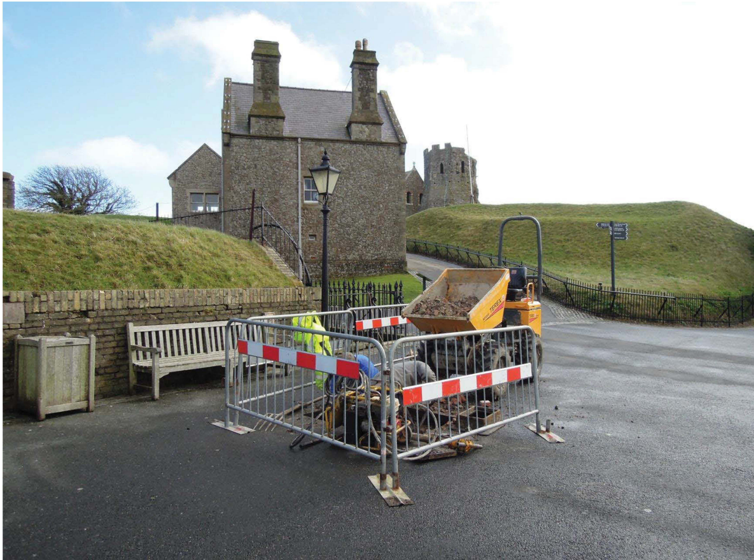
Plate I General view of Pit 2 in Harold's Road, looking south-east
