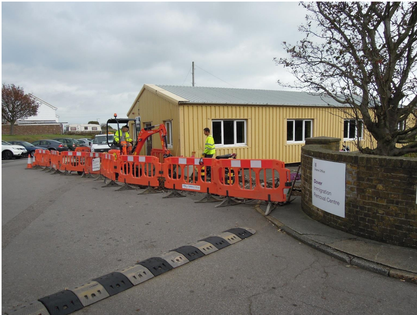
Frontispiece Trenching in progress at Site 2 (Visitors Centre), looking north-east
