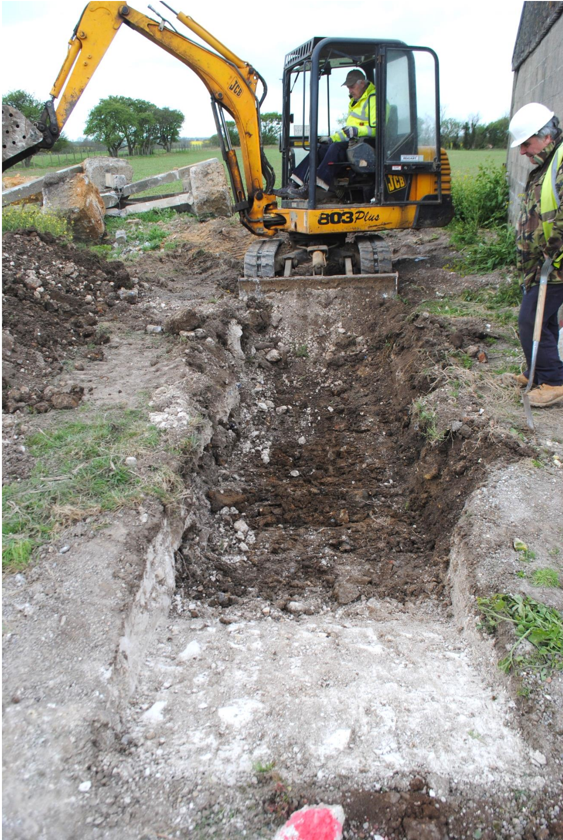
Frontispiece Machine excavation of Trench 2, looking west
