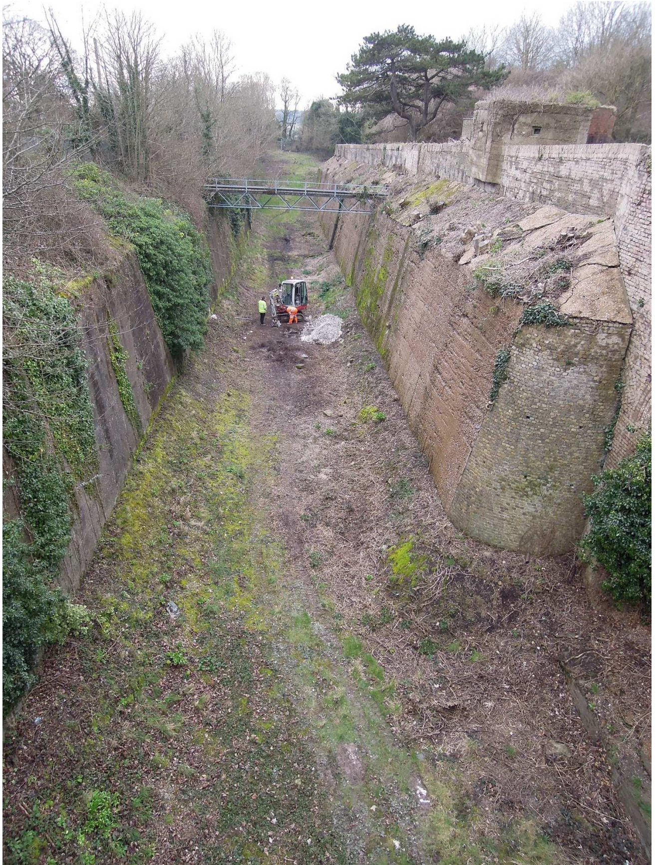
Frontispiece Machine excavation of Test pit1 in the ditch, looking west
