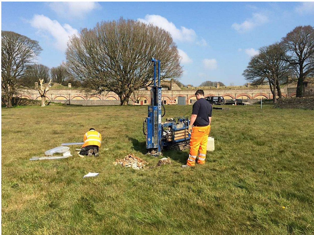
Fig. 6 Drilling Borehole 3, looking north
