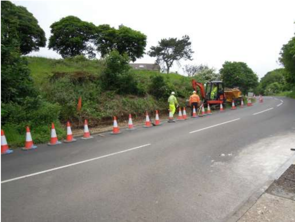
Plate IV Footpath along western side of Centre Road under construction, looking north
