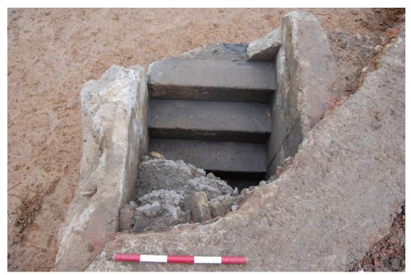
Plate 56. G31 air-raid shelter \$5291 showing concrete entrance stair-way, looking north-east (scale 0.5m)
