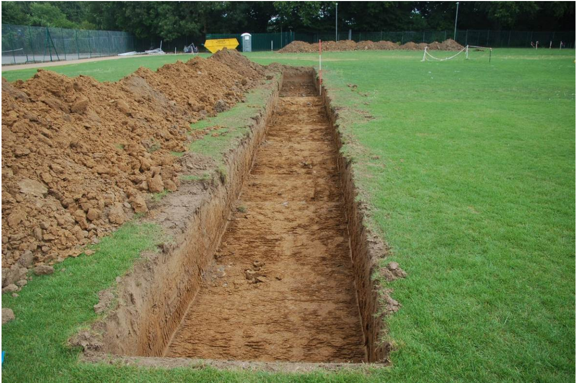
Plate 3. Trench 2 looking south-east (scale 2m)
