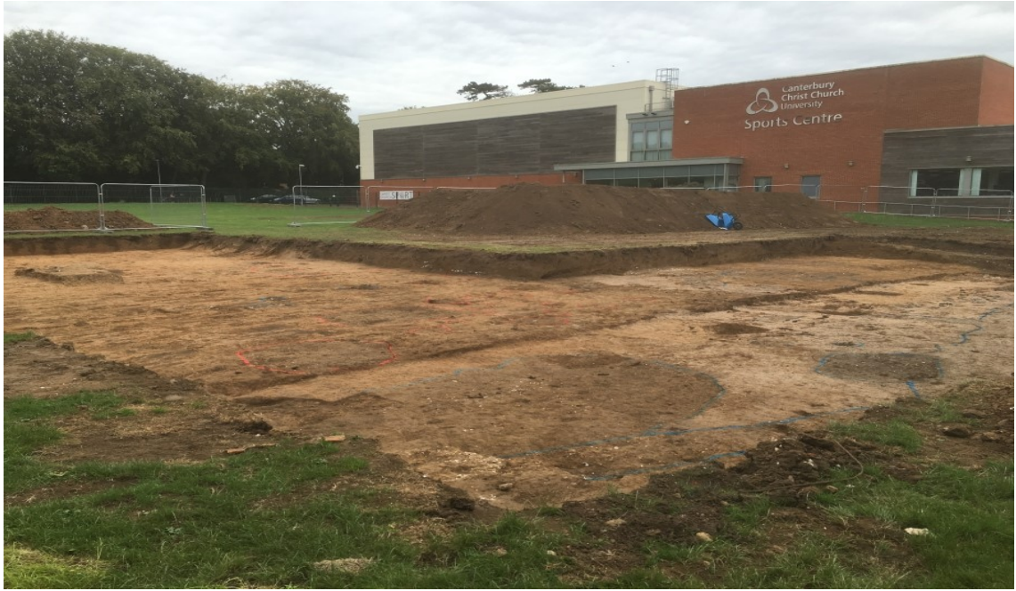
Plate 10. Excavation area looking south-east
