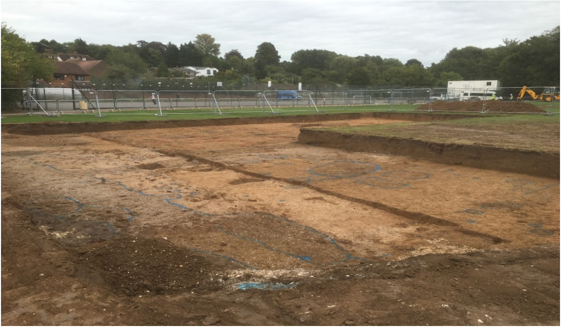
Plate 8. Excavation area looking north-north-east
