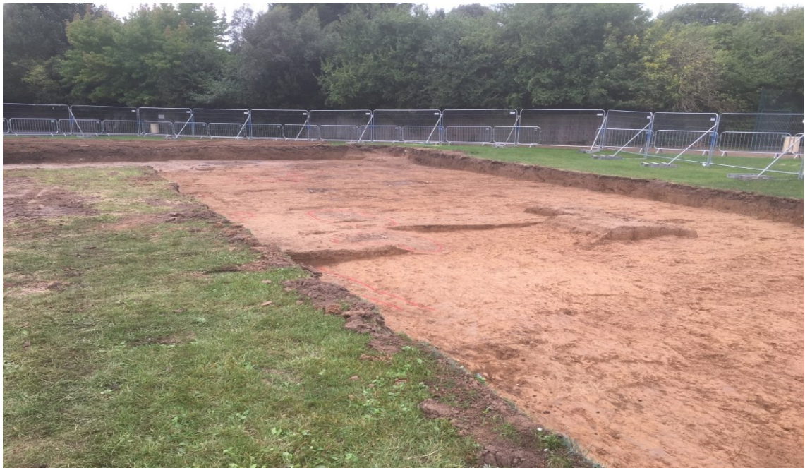
Plate 11. Excavation area looking west
