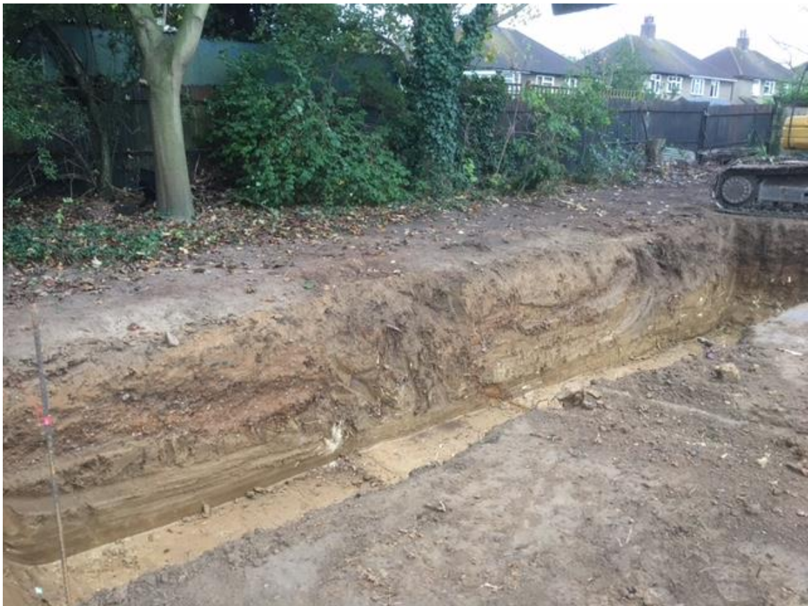
Plate 4: Excavation for attenuation tank 1 looking south-west
