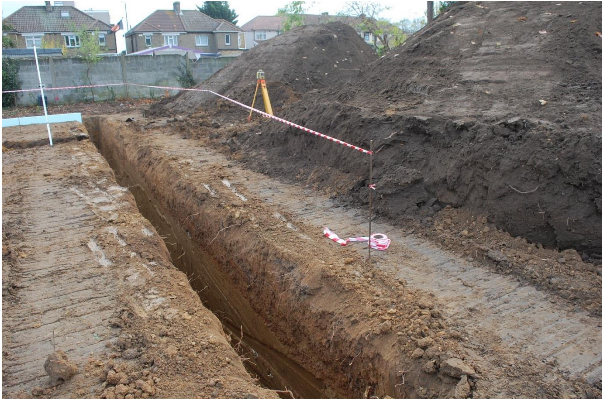
Plate 9: foundation trench of block 'C' looking north-east
