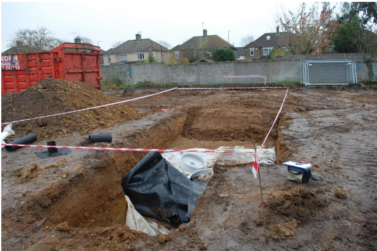
Plate 6: Excavation for attenuation tank 2 looking east
