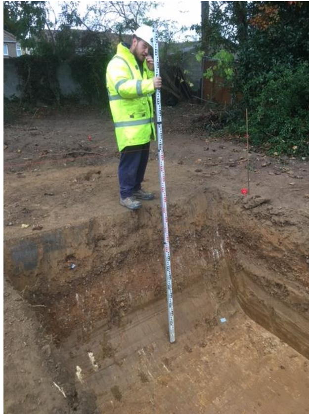
Plate 5: Section of attenuation tank 1 excavation looking south-east.
