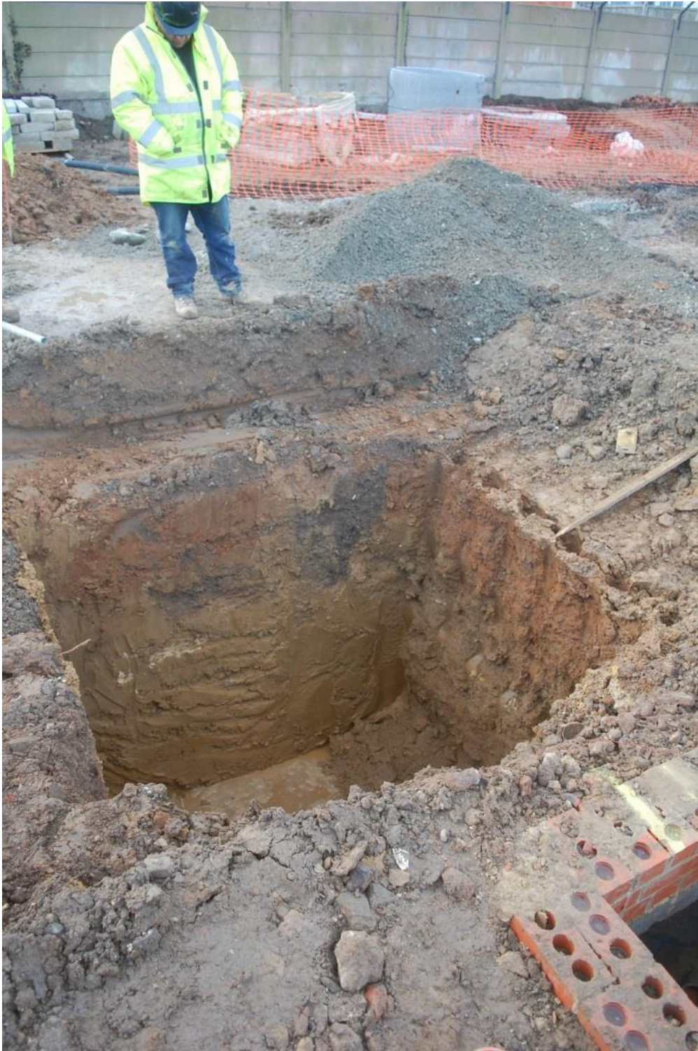
Plate 11: Pump station pit looking west
