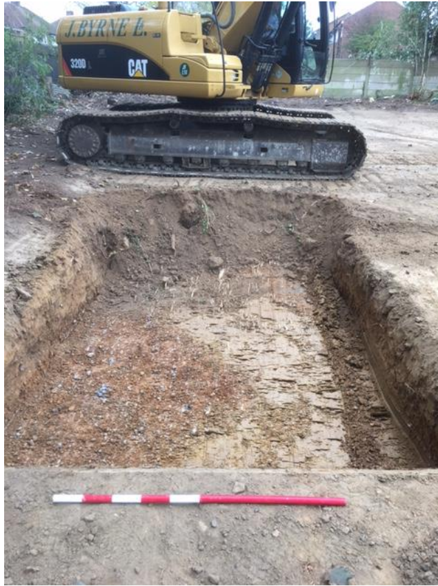
Plate 3: Excavation for attenuation tank 1 showing gravel layer (1005) looking west. Scale 1m
