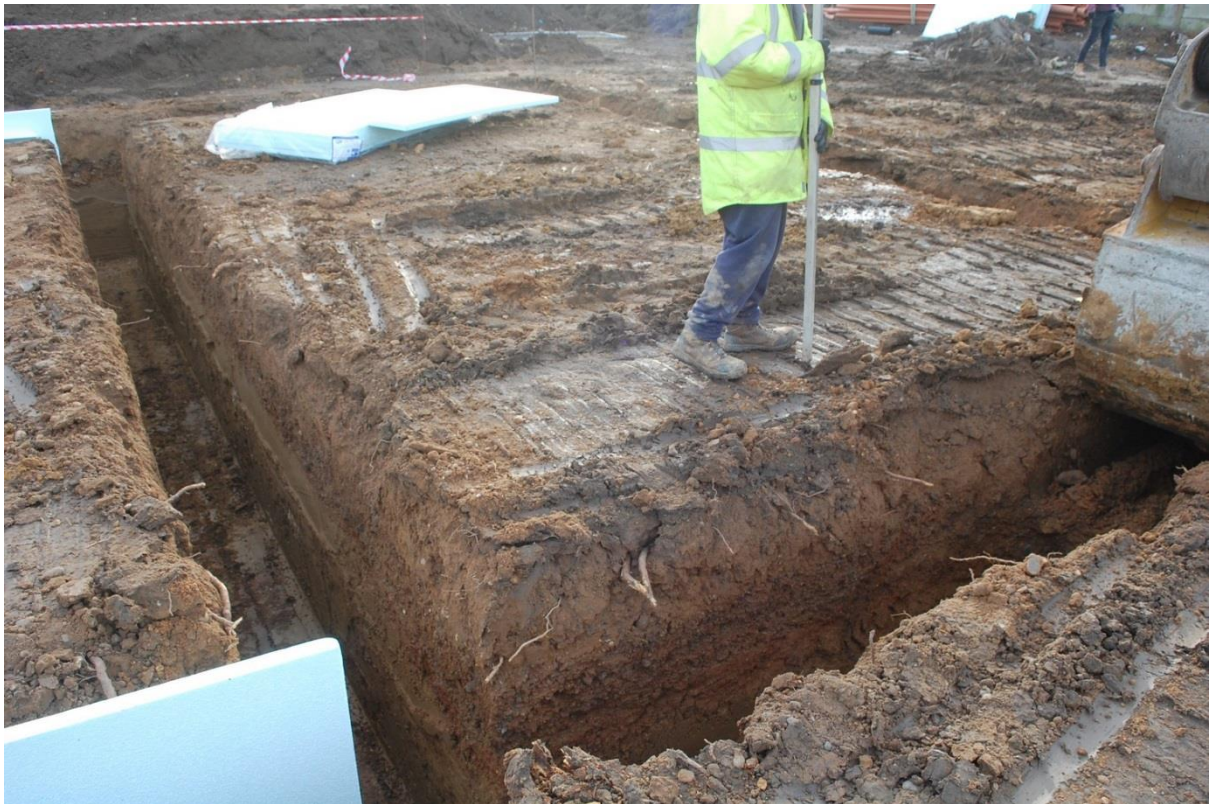
Plate 10: foundation trench of block 'C' looking south-west
