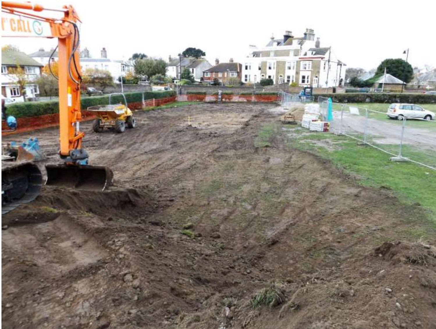
Frontispiece General view of earthmoving on site, looking west (CAT image 3474)
