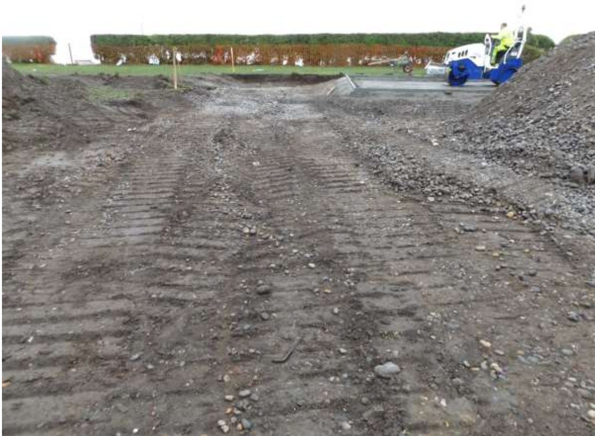
Fig. 11 Excavations for the car park, looking east (CAT image 3440)
